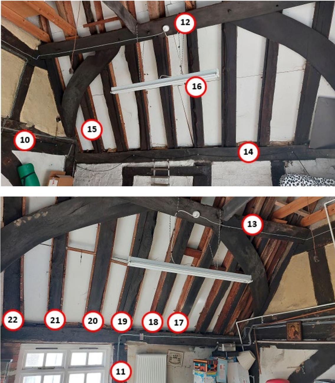
Figure 4a/b: Annotated photographs of the roof over the south bay to help identify sampled timbers, looking east (top) and west (bottom). [photographs Robert Howard]
