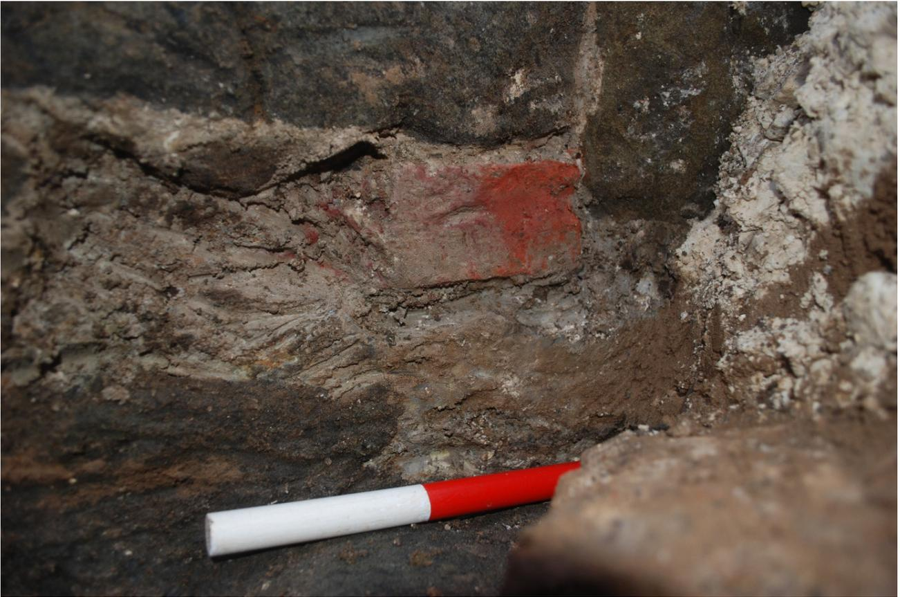
Figure 9: Detail of post-medieval brick and cream lime mortar.
