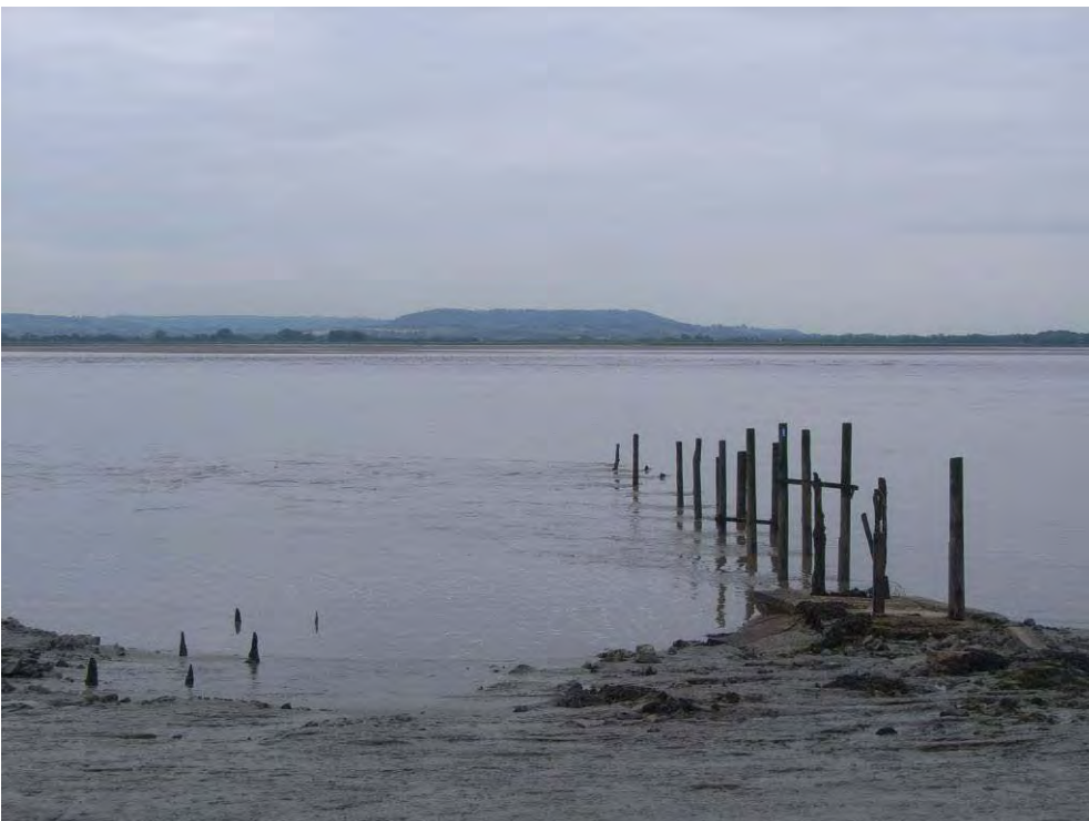
Plate 150: Two putcher ranks south of Awre, Glos, with a modern putcher rank on the right ( Line No. 10064 ) built of telegraph poles, metal joists and concrete that replaced an earlier all-wooden putcher rank visible on the left ( Line No. 10065 ).
