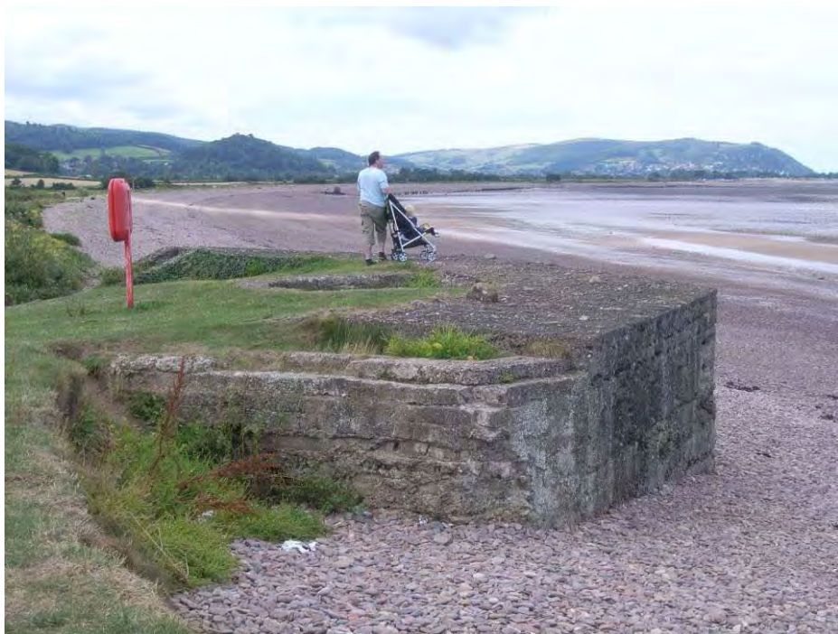
Plate 262: The rare surviving infantry section post at Blue Anchor Bay, Som. ( Point No. 3009 ). The emplacement on its roof was for an anti-aircraft gun, though few were ever fitted.
