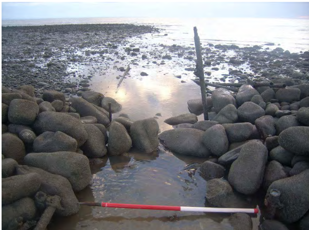
Plate 28: The gut or outflow channel of a stone fish weir at Warren Point, east of Minehead Bay, Som. (Line No. 10204). Note the metal scaffolding poles.
