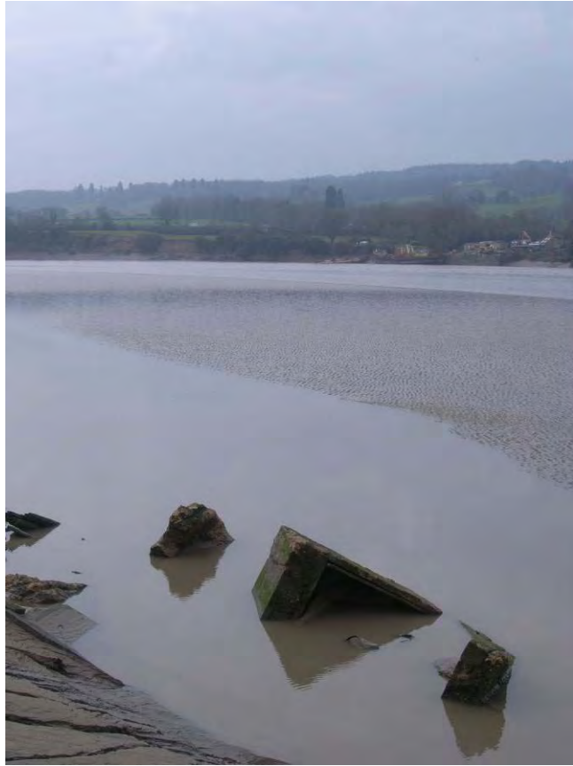
Plate 261: The pillbox near to the Old Passage Inn at Arlingham ( Point No. 118 ) has slipped off the riverbank completely and is now in the active river channel, being buried by river silts.
