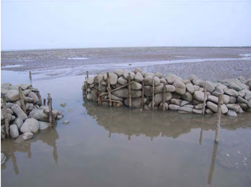
Plate 31: Another well-defined apex and gut on a stone fish weir at Minehead Bay, Som. (Line No. 10381), where metal scaffolding poles have been used as revetment for the stone walling as well as to support catch baskets or nets.
