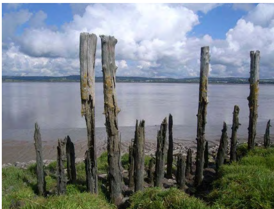
Plate 244: Eroded coniferous wooden posts of relatively recent date north-east of Severn House Farm, Ham & Stone, Glos. ( Line No. 10106 ), possibly some form of revetment structure.
