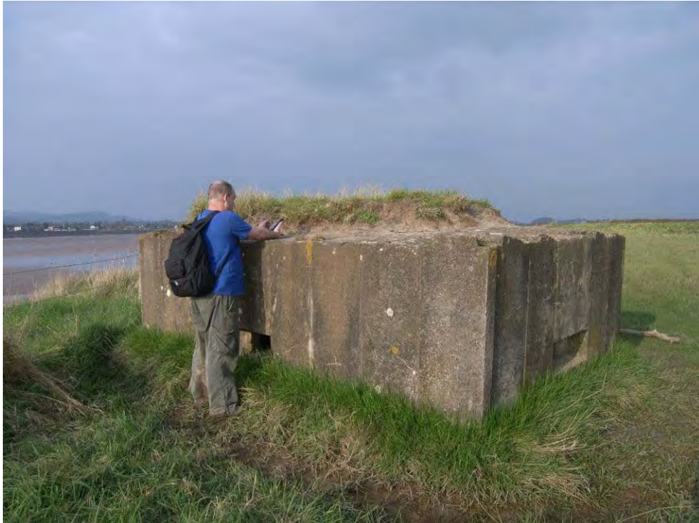
Plate 259: Toby Catchpole recording a pillbox north of Passage Farm, Arlingham, Glos. ( Point No. 123 ). Although well-preserved, the entire structure is slowly sinking into softer underlying alluvial deposits.
