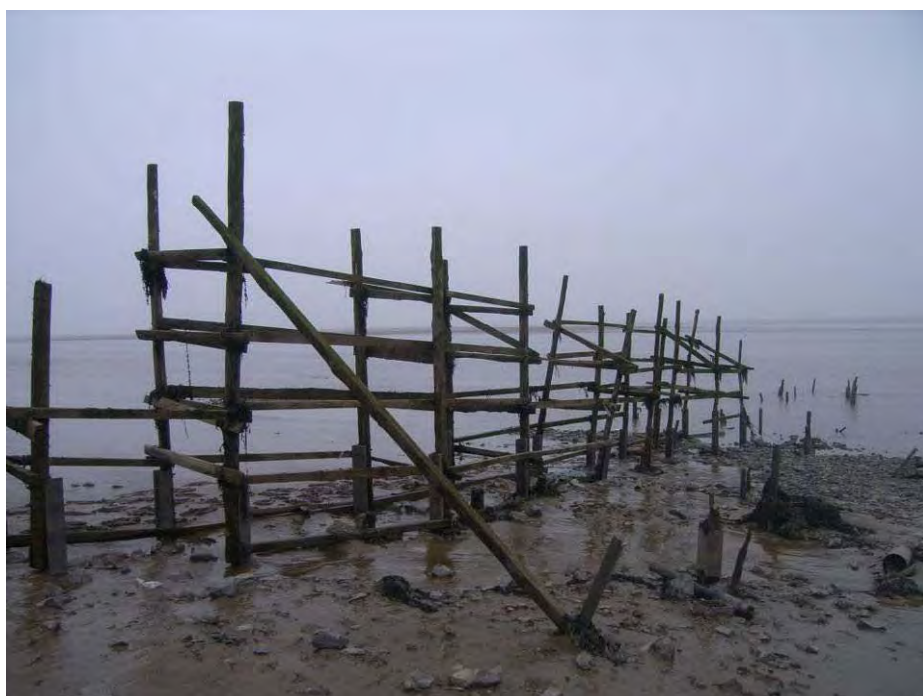
Plate 148: A 20 th century putcher rank south-west of Brims Pill, Awre, Glos. ( Line No. 10350 ), with horizontal basket supports, metal pipes and downstream bracing timbers.
