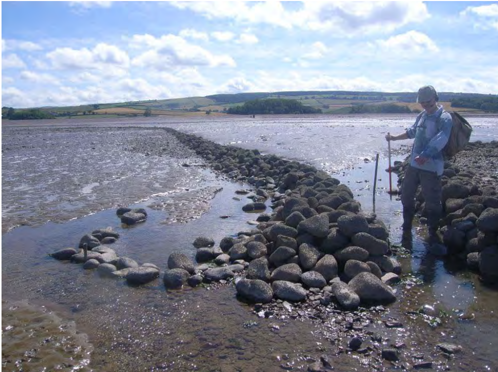
Plate 43: Richard Brunning examining the well-built gut or outflow channel from a stone fish weir still in use at Blue Anchor Bay, Som. ( Line No. 10145 ). Note too the appended L-shaped structure.
