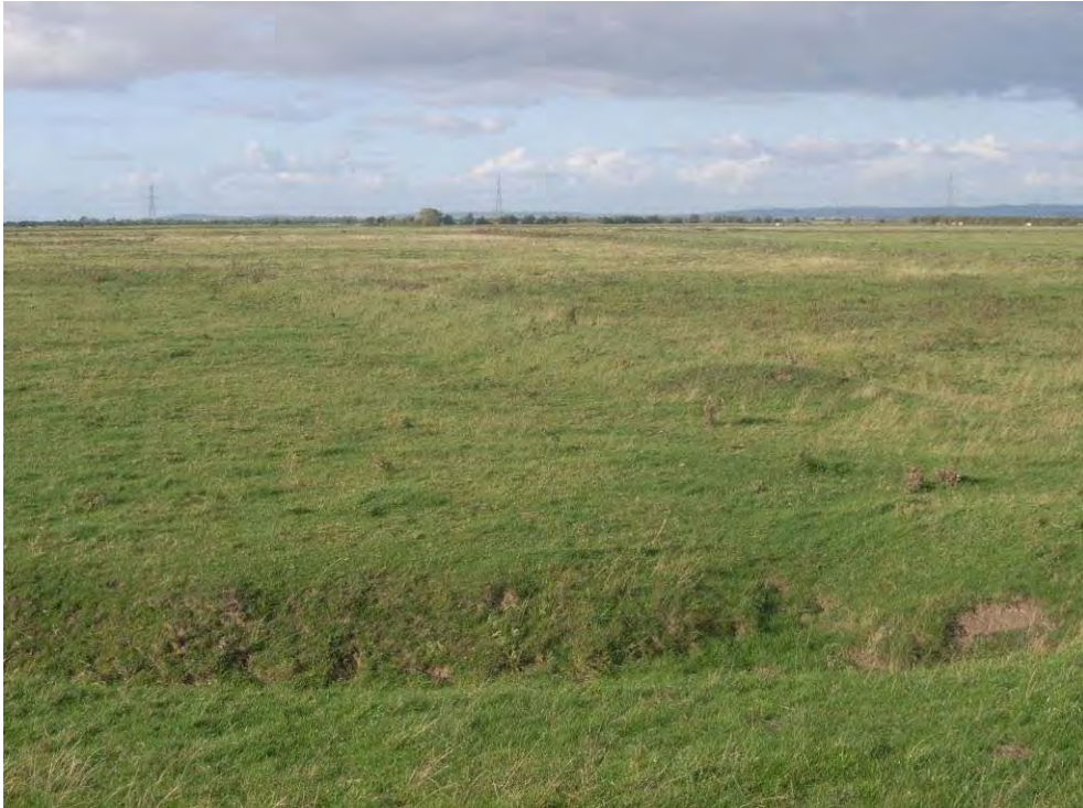
Plate 251: Earlier phases of flood defence near at Pawlett Hams, Som, taken from the existing defence bank. One back scarp ditch can be seen in the foreground, whilst an earlier bank extends from the mid-right to the upper left of the image. Not formally recorded.
