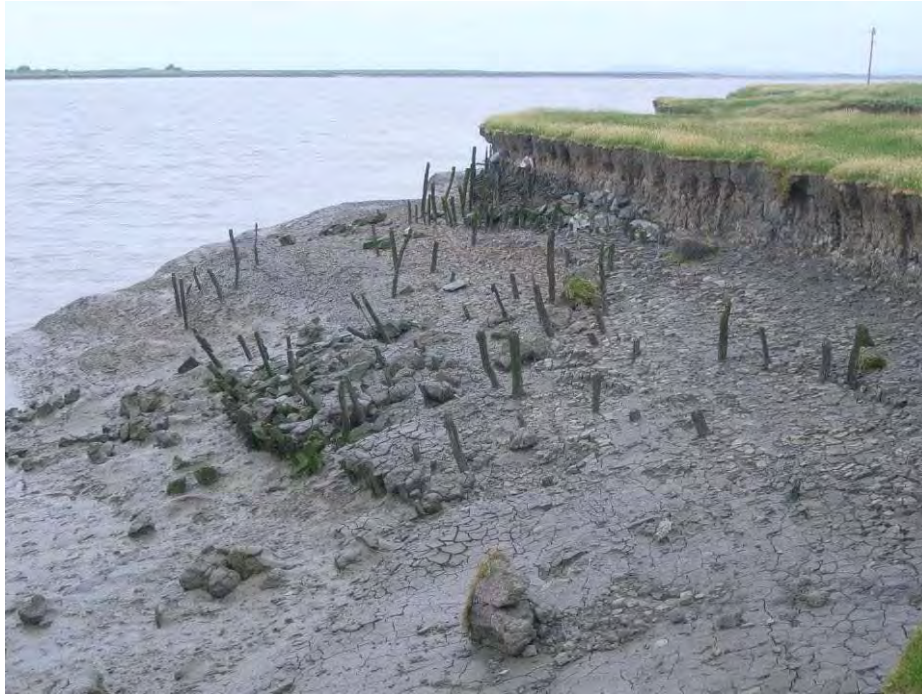
Plate 241: Several different phases of riverbank revetment or cribbing at Stockland Reach, Pawlett Hams, Som. ( Line No. 10001 ).
