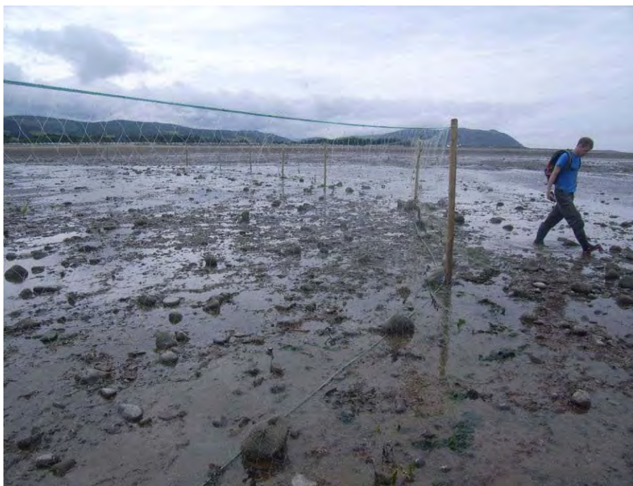
Plate 8: A contemporary net hang line still in use at Dunster Beach; illustrating its construction with wooden posts and beach boulders as footrope weights ( Line No. 20038 ).
