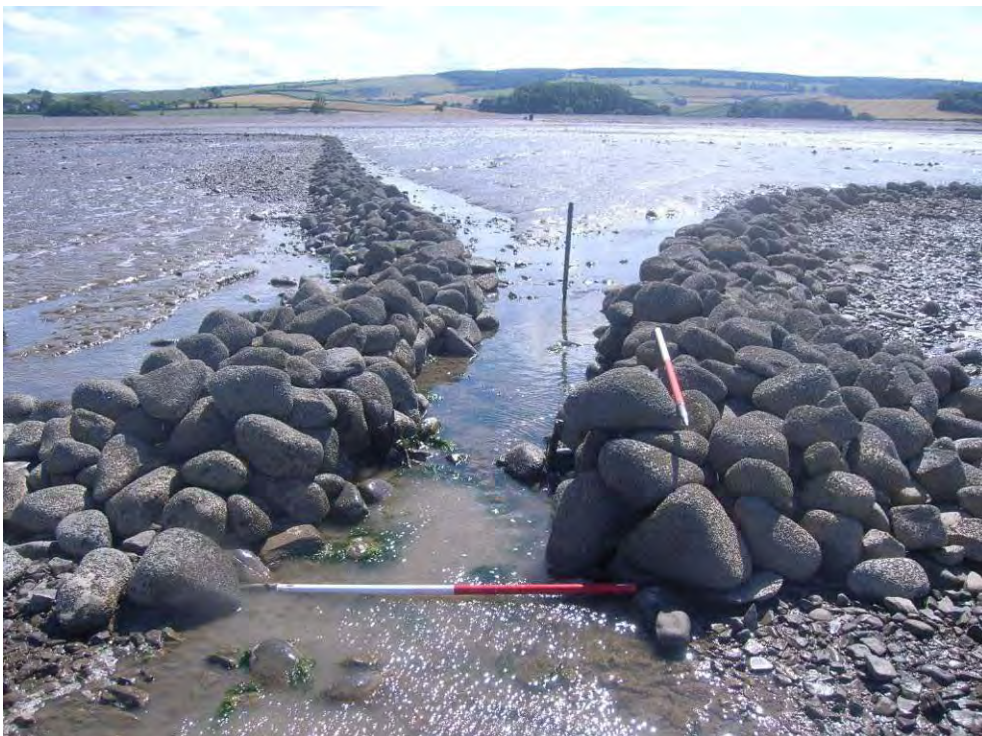
Plate 22: The apex and outflow channel or gut of a large stone fish weir at Blue Anchor Bay, Som. ( Line No. 10145 ), part of two conjoined and contiguous examples. This well-preserved structure with metal poles may still be in occasional use.
