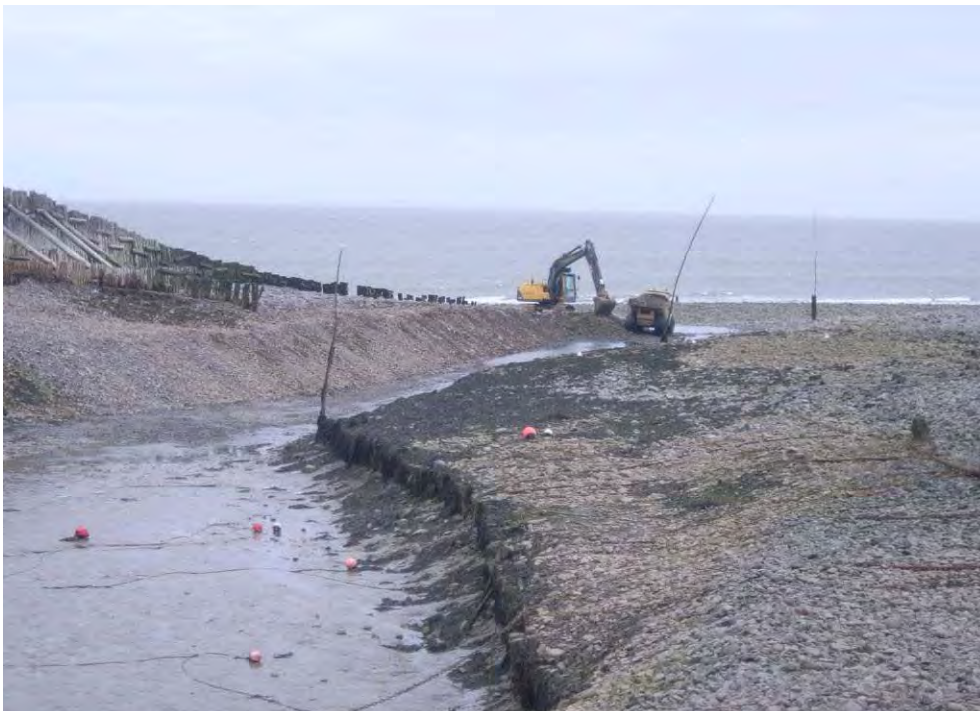
Plate 298: Large earth-moving plant being used to machine out the channel leading to the harbour at Porlock Weir, Som. in 2009. Such groundwork should always be subject to archaeological mitigation, including the possibility of watching briefs and evaluations.
