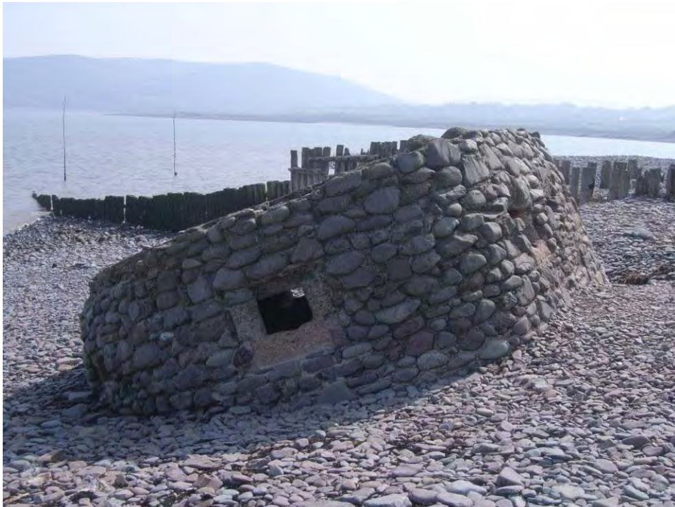
Plate 258: One of two camouflaged pillboxes at Porlock Weir, Som. This example is subsiding and tilting down into the softer underlying shingle and pebble beach. It was not formally recorded.
