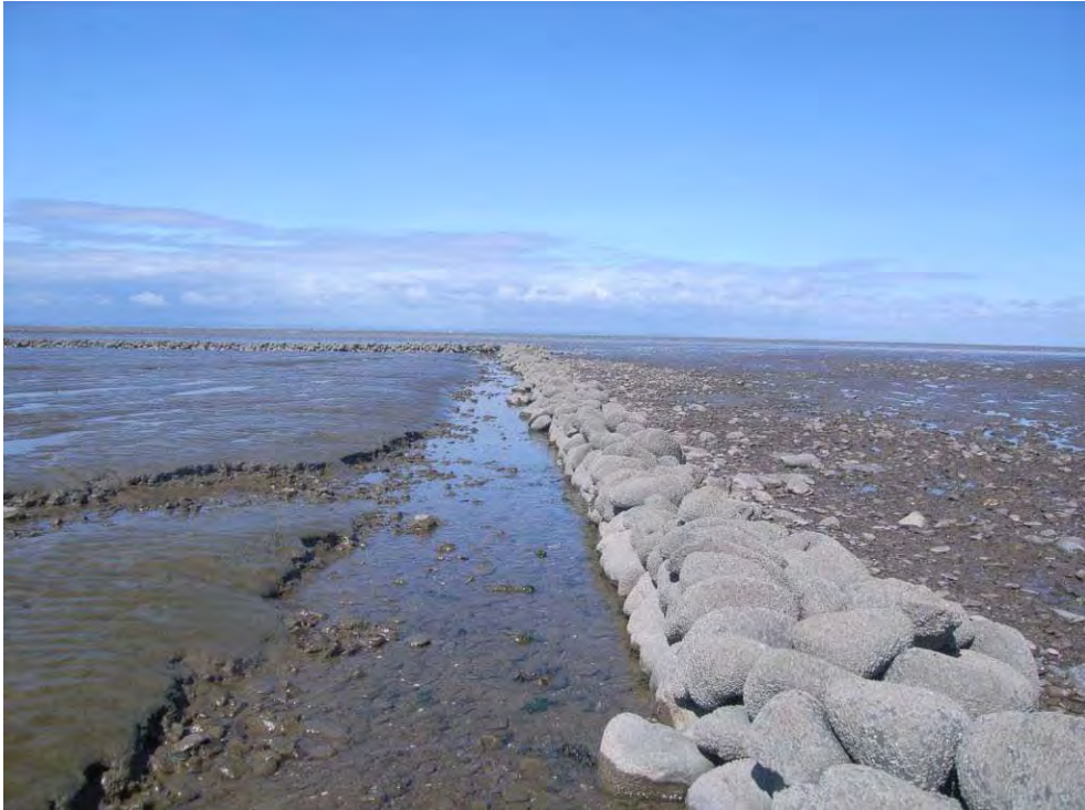
Plate 35: One of the leader arms of two large, V-shaped stone weirs forming a contiguous structure at Blue Anchor Bay, Som. ( Line No. 10145 ), which is still used and maintained.
