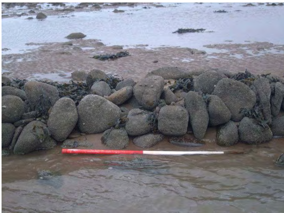
Plate 34: The leader arm of a well-built stone fish weir constructed of cobbles in a 'drystone wall' pattern, Minehead Bay, Som. (Line No. 10190).
