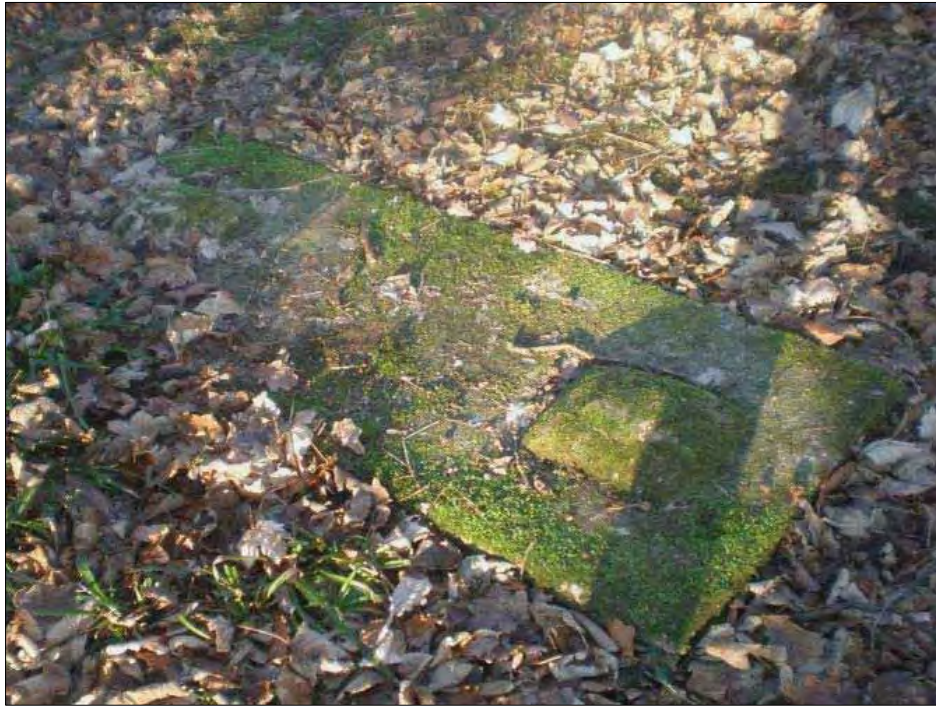
Figure 3.14 Example of a concrete footing for the (now removed) over-ground pipe network. These are located throughout the north and east of the enclosure.
