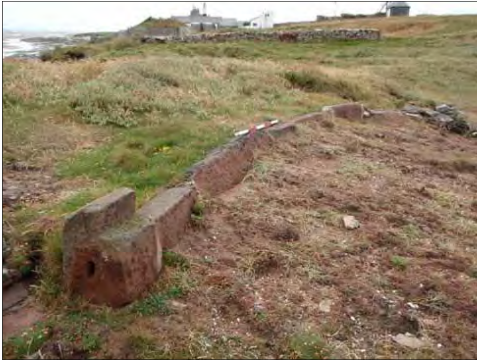
Figure 3.3 Re-used punched-dressed sandstone masonry with part of a door jamb in the foreground. (scale=1m).
