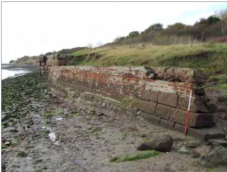
Figure 3.19 Remains of red sandstone and brick wharf looking west (scale = 1m).
