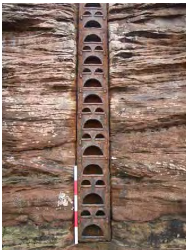
Figure 3.6 Iron steps recessed into the cliff-face to the east of the lifeboat station (scale = 1m).
