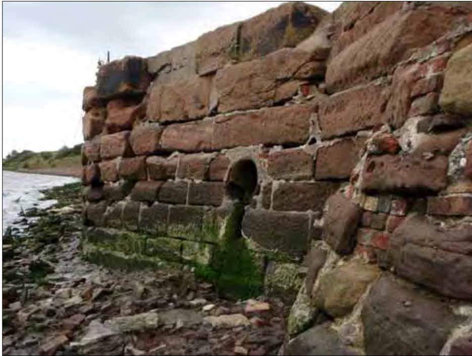
Figure 3.20 Dogleg in the course of the wharf, possibly indicating the juncture between two phases of construction. Looking west
