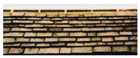
Figure 15 'Pigs' (where a long margin is visible above a short one) indicate a failure to maintain adequate head lap and are evidence of poor workmanship, as this roof in West Yorkshire shows.
