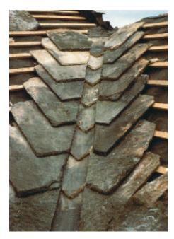
**Figure 12** The heavy, flat sandstone flags of the South Pennines are suitable for lower pitches, and the detailing of the roof is simpler to accommodate their large dimensions. The chevron valley is an example of the craftsperson's skill in forming a weather-tight roof.
