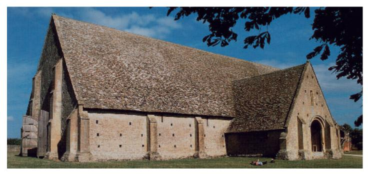
Figure 19 These small Cotswold stone slates have been laid at a steep pitch to form the huge roof of Great Coxwell Barn, Oxfordshire.
