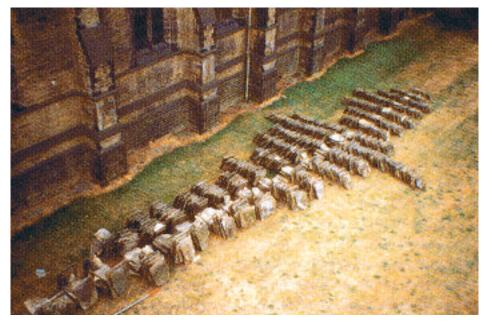
Figure 8 Stone slates removed from the roof and sorted according to size. The roofer will now be able to calculate the amount of new material required for reroofing.
