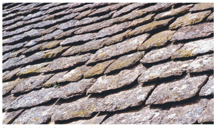
Figure 16 Langley Chapel, Shropshire. This Harnage stone slate roof includes both sandstone and calcareous sandstone, which overlie each other in the same quarry. The calcareous sandstone is identifiable by the presence of white lichen.
