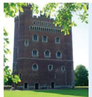
Figure 10 Luminescence dating of known age buildings, such as Tattershall Castle, Lincolnshire (shown here), to assist in the development of this technique. The independent date range for the sampled part of the building was AD1445-1450, luminescence dates were 1455  $\pm$  33 and 1455  $\pm$ 34. Image and data courtesy of lan Bailiff.
