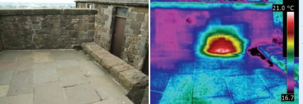
Figure 12a Left Figure 12b Right Heat from a concealed flue in a parapet wall. The flue from the chimney of the kitchens at Stirling Castle has been blocked up and covered, with the area above becoming used as a parapet. However, heat rising from the flue is still visible to thermal imaging. Images by Maureen Young, Historic Scotland.
