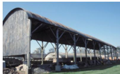
Dutch barns were first built of timber and corrugated iron, and then a mixture of timber, iron and steel frames. They became standardised from the 1880s when firms began to advertise and issue printed details with drawings, usually along with other 'kit buildings' such as parish halls. Photo © Joan Grundy
