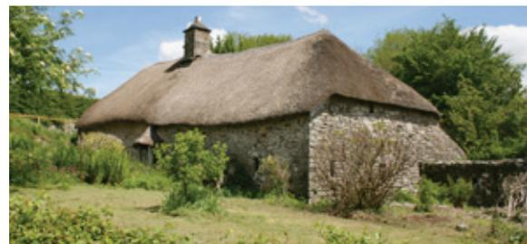
Higher Uppacott at Poundsgate. The early 16th century longhouse is built into the sloping ground, and the photograph shows the ventilation slits to the well-preserved lower shippon end which retains its central drain. Photo © Dartmoor National Park Authority
