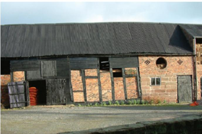
Successive phases of rebuilding are a key characteristic of vernacular farm buildings in particular. This timber-framed building in the Cheshire Plain had its wattle and daub infill replaced by brick in the 19th century, and was also then extended in sandstone blocks and brick. Corrugated iron, used from the 1820s for industrial buildings, was commonly used for repairing roofs by the First World War. Photo © Jen Deadman
