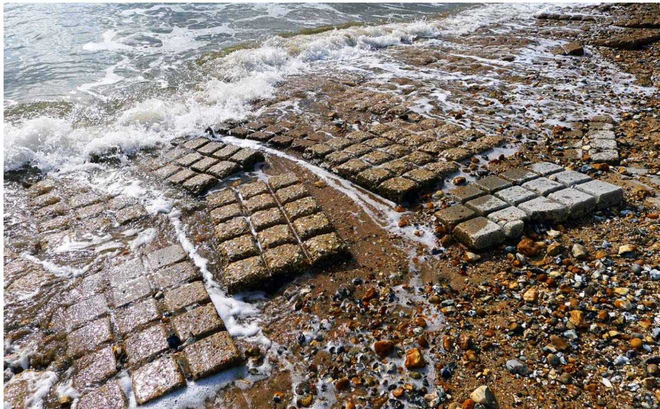
Above left: Stokes Bay, concrete matting laid to assist troop embarkation for D-Day. Photograph courtesy W D Cocroft
