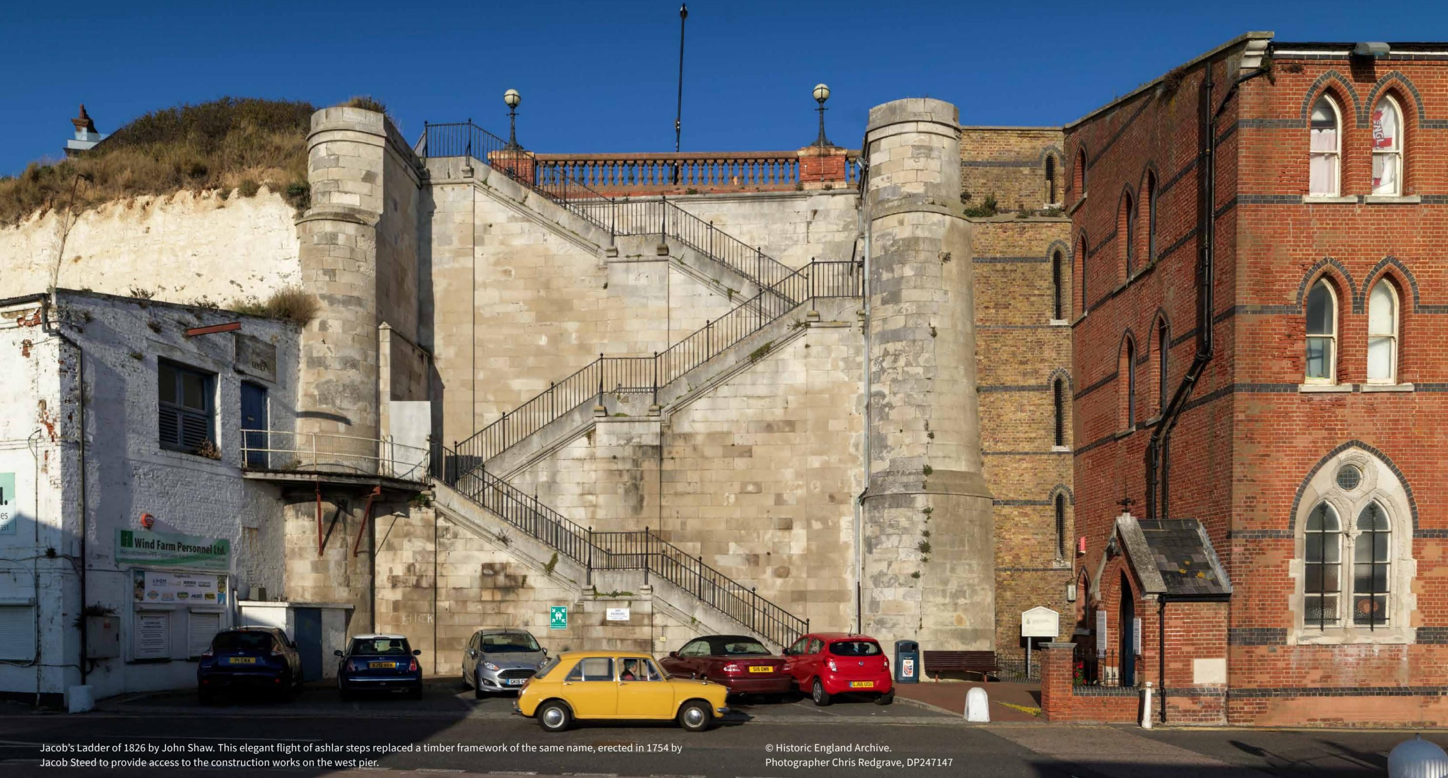
Jacob's Ladder of 1826 by John Shaw. This elegant flight of ashlar steps replaced a timber framework of the same name, erected in 1754 by Jacob Steed to provide access to the construction works on the west pier.
