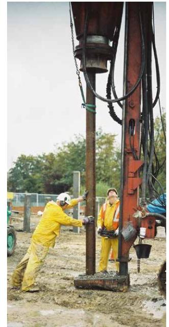
Figures 11 and 12: Sheet pile retaining wall along the edge of a site at Drapers' Gardens (left) © Pre-Construct Archaeology Ltd. Rolled steel tube being installed at Skirbeck Road, Boston (right).
