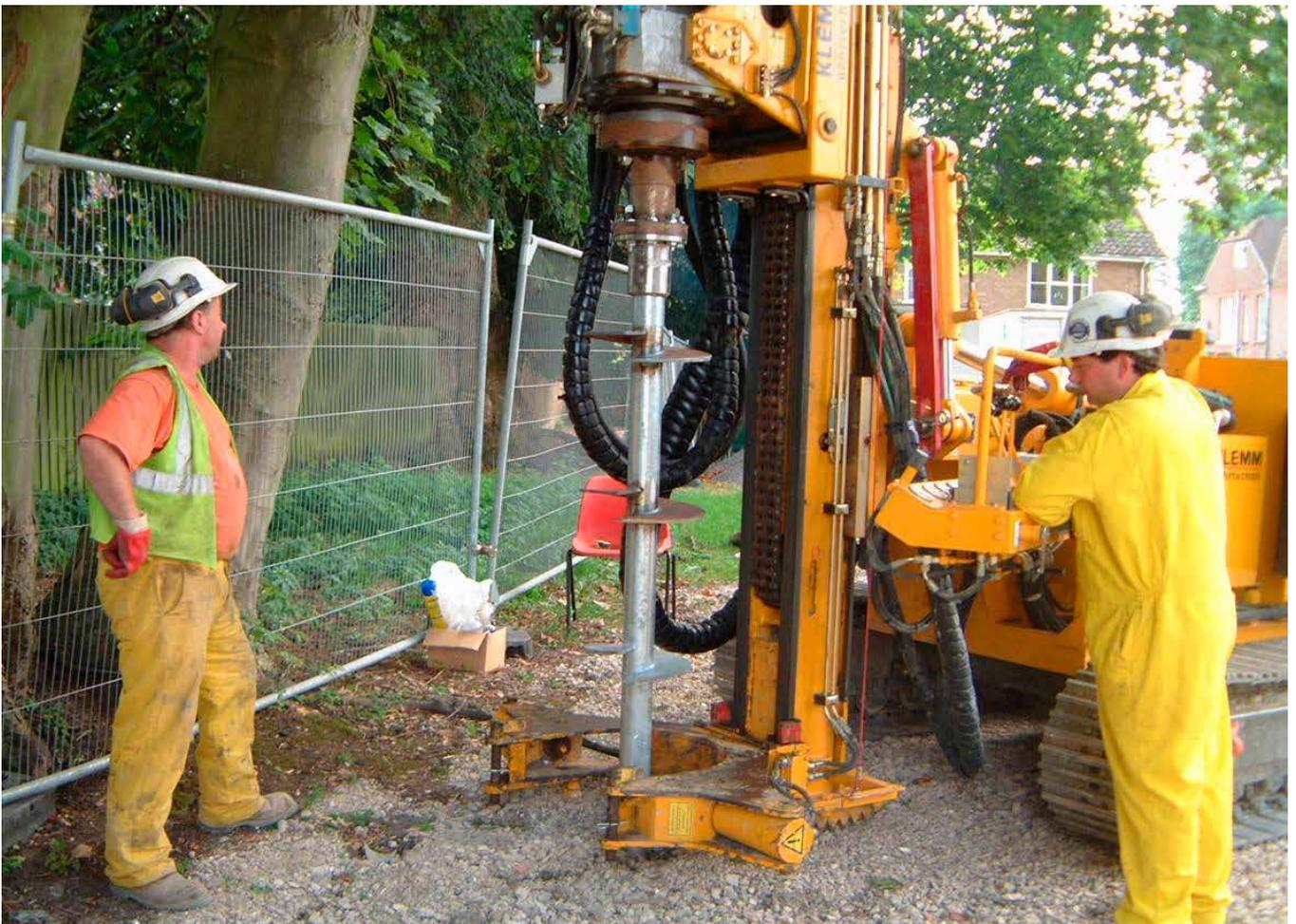
Figure 36: Screw piles being installed. © Tim Sheward
