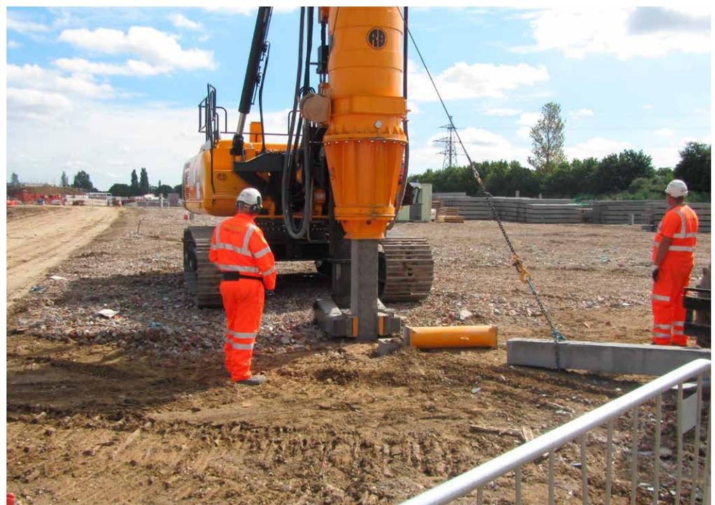
Hollow piles are tubes generally constructed of steel or occasionally precast concrete. The concrete may be pre-stressed to enhance durability. Hollow piles are often used when large diameters (>500mm) are needed and are hollow for ease of handling, or for economy. For hollow steel piles, concrete is poured into the hollow section to complete the pile (as for driven cast *in situ*), except that in this case the tubes are not withdrawn.
