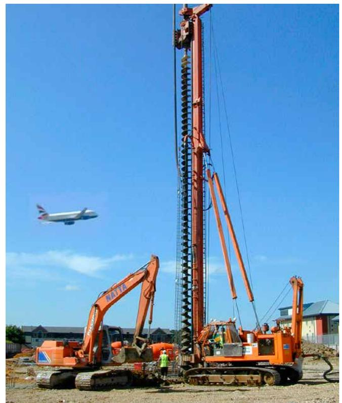
Figure 17: Continuous Flight Auger (CFA) piling. © Cementation Foundations Skanska
