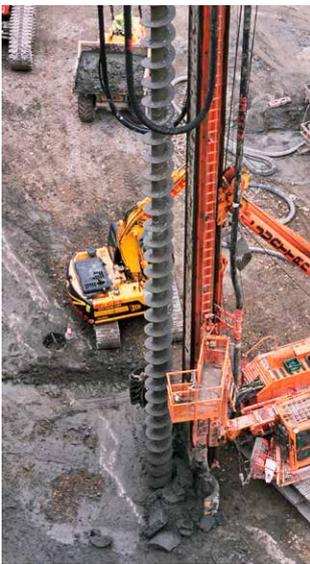
Figure 15: Photograph from above a CFA pile during the construction of a pile. Soil can be seen in the lower flights, and around the auger where it has been cleaned off. The reinforcement cage stands adjacent (left). © Cementation Foundations Skanska
