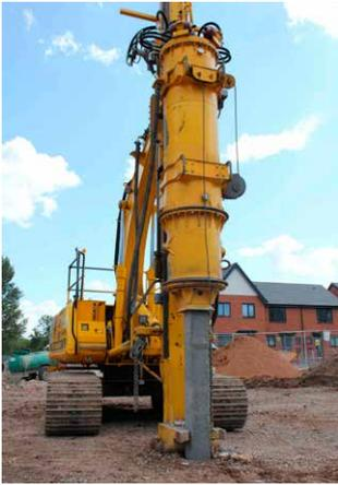
Figure 7: Preformed concrete displacement pile being installed.
