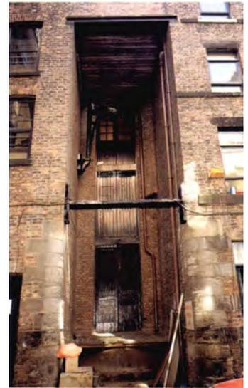
*Fig 30 (opposite, top) Teagles and goods doors at the rear of 70–2 Portland Street (compare with the front elevation in Fig 29). [AA026864]*
