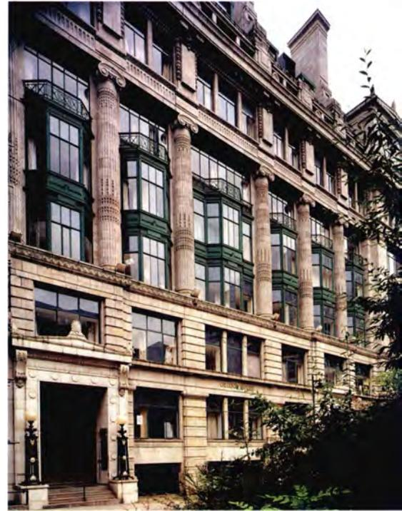
*Fig 9 Orient House, 65–7 Granby Row, was a packing warehouse for Barlows Ltd, a makers-up firm and packing company. It was designed by Henry Goldsmith and built in 1912–16. The fine frontage contrasts with the purely utilitarian rear and sides. [AA022619]*
