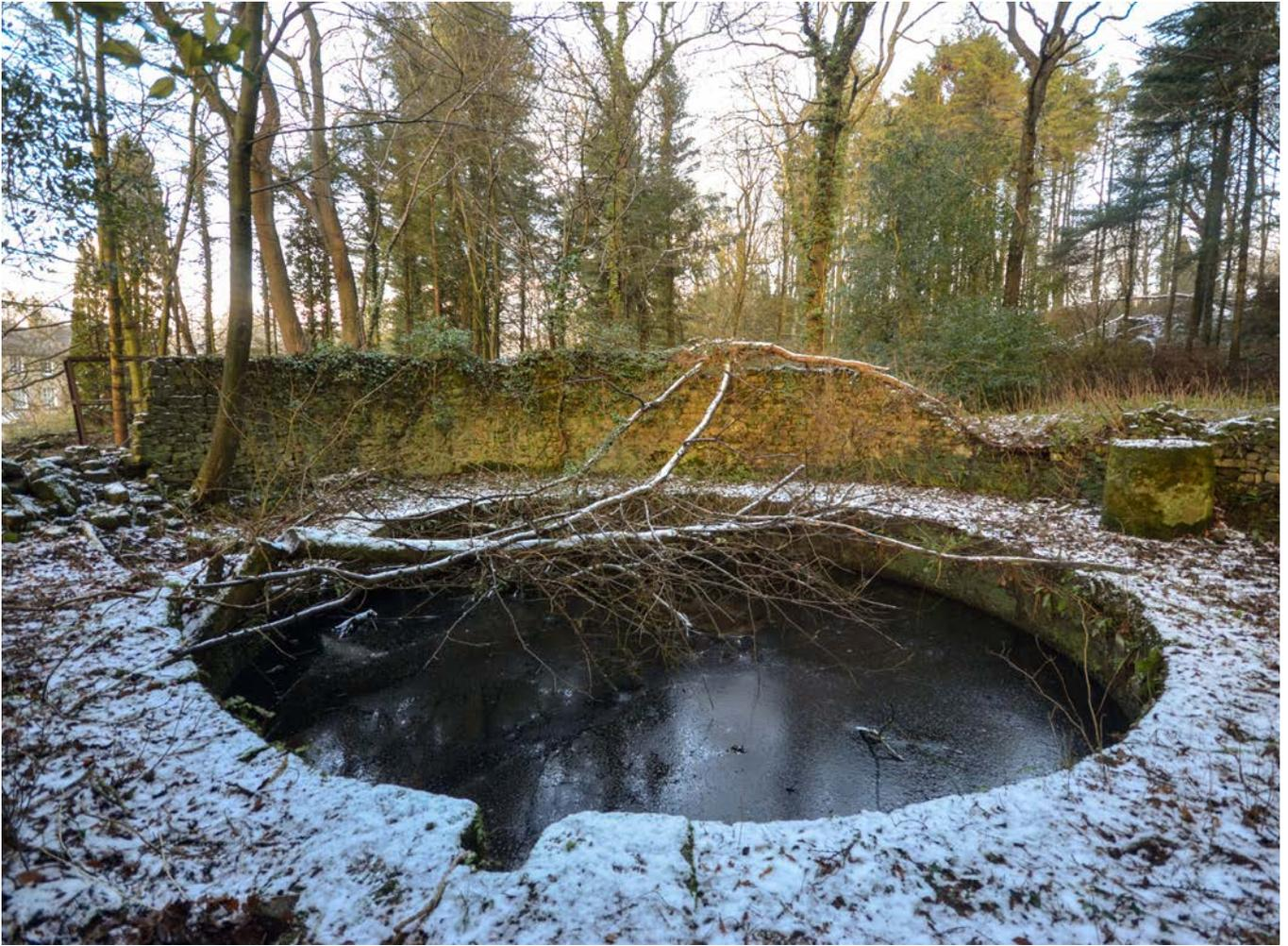
Figure 1: The surviving tank of a gasholder built in about 1820 at Dolphinholme worsted mill by the pioneering gas engineer, Samuel Clegg. The location of the stanchions which formerly supported the bell remains clearly visible, while the large stone counter-weight is a unique survival.
