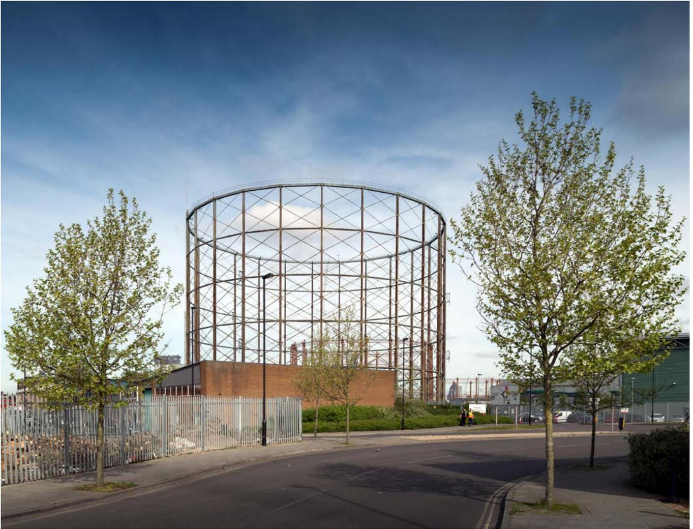
Figure 10: Gasholder No.13, Old Kent Road, Southwark, London (Built 1879-81 and listed in 2017). With exceptionally thin wrought-iron standards (uprights) linked by girders and diagonal struts this pioneering gasholder essentially forms a three-dimensional cylindrical shell. It inspired the development of helical or geodesic structures. The bell used mild-steel for the first time, and the innovative tank was the deepest then constructed and one of the deepest ever built. [DP182523]
