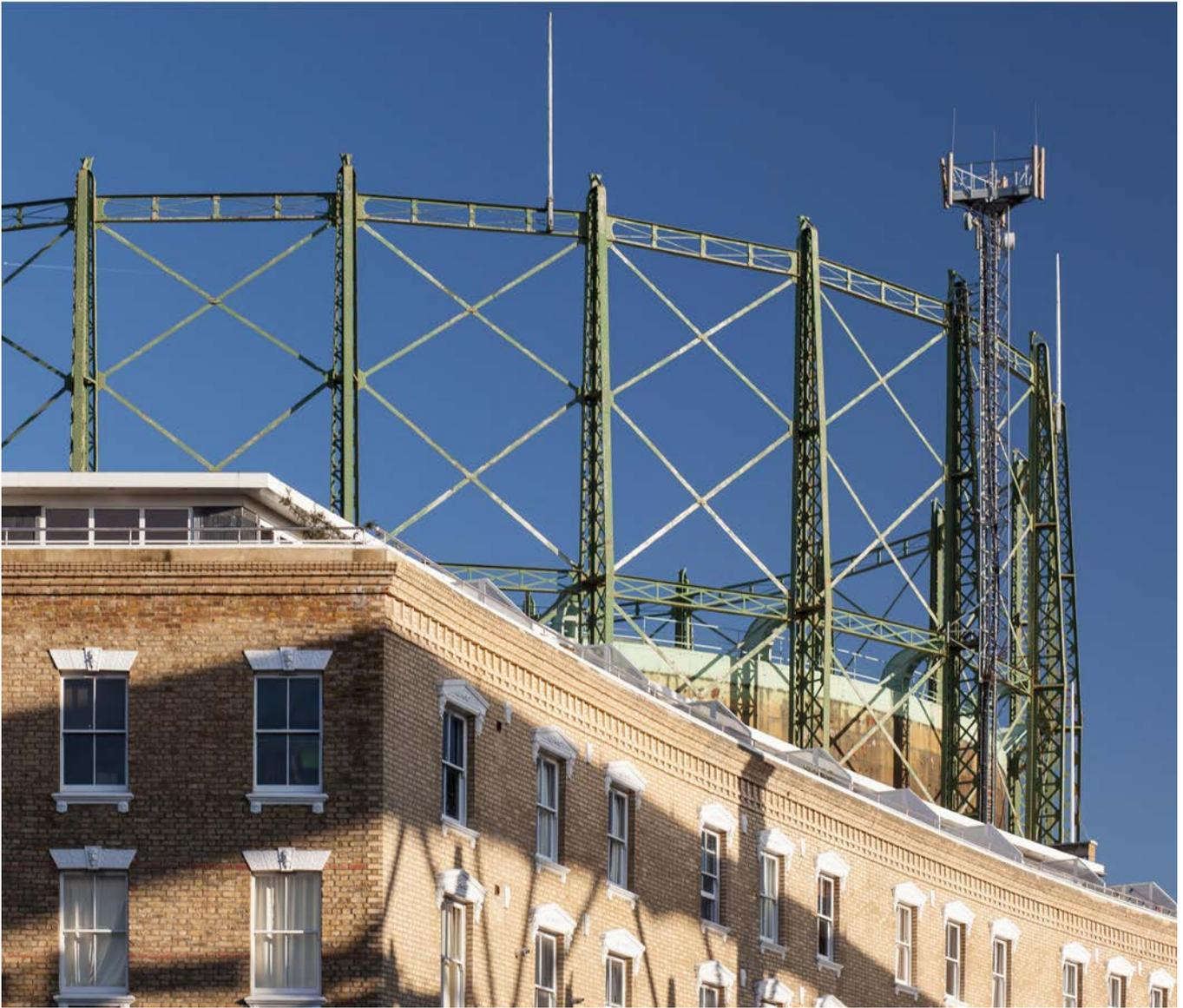
Figure 9: Gasholder No.1 adjacent to The Oval cricket ground, Kennington, London (Built 1877-79 and listed in 2016). Note the wrought-iron lattice standards (uprights), cross girders and diagonal-bracing of the guide frame. The telescopic bell is partially-filled, rising just above the building in the foreground. [DP182564]
