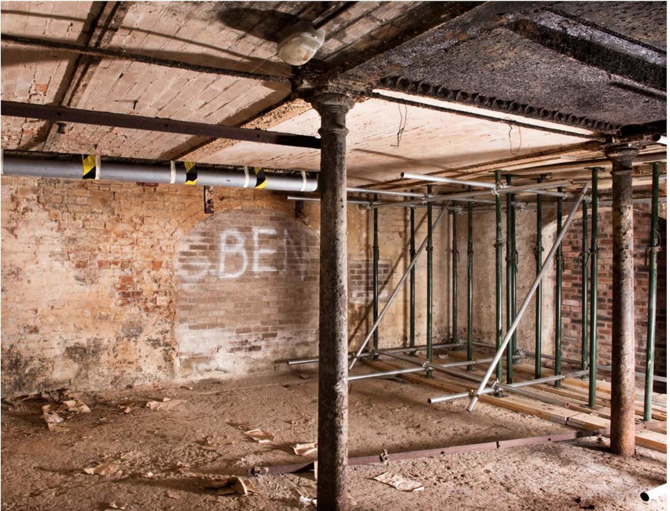
Figure 13: Interior view of the ground floor of the former purifier house at the Gloucester Gaslight Company's first gas works on Quay Street, Gloucester. Constructed in the early 1850s to house dry lime box purifiers, the building was designed to be fireproof and was constructed around two arcades of cast iron columns which carried cast-iron girders and a ceiling of brick jack arches and cast iron plates. It was demolished in late 2017. [DP219975]
