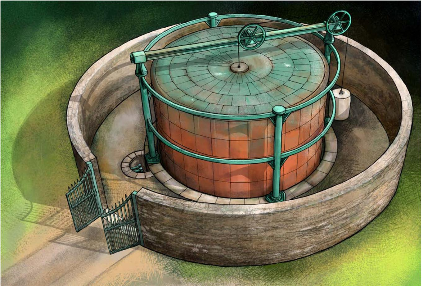
Figure 6 (top): The gasholder at the former Dolphinhholme Worsted works as it may have looked in around 1820 after its construction following a major extension of the mill in 1818. The remains of the holder, comprising the circular stone tank, rubble stone wall and counterweight form part of what is thought to be the world's earliest surviving gasworks. © Historic England
