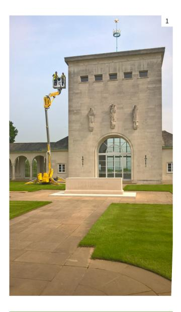
**Figure 1**Access platform for inspection, Runnymede Memorial, which is in the care of the Commonwealth War Graves Commission.
