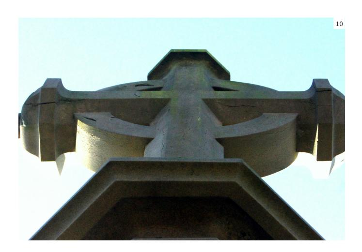
Figure 10 Cracking beyond fingertip reach recorded by telephoto lens, Southborough War Memorial, Kent.
