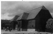
*Water reed thatch at Wimpole, Cambridgeshire, showing the exactness with which this material takes up the lines of the roof*
