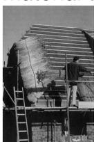
*Water reed thatching in progress on a new roof structure. Particular care is taken with the eaves, as in all thatching*
