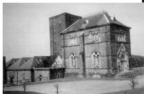
*Dalton Pumping Station: this Grade II\* complex was one of a series designed by Thomas Hawksley to supply drinking water from the Durham aquifers to the towns of Tyneside and Wearside. The massive engine house in brick and stone with its grand entrance, arched windows, and wall buttresses, still retains much of its original – if now, non-functioning – machinery. Grant aid will return the building and its fittings to a stable condition in preparation for an appropriate new use*
