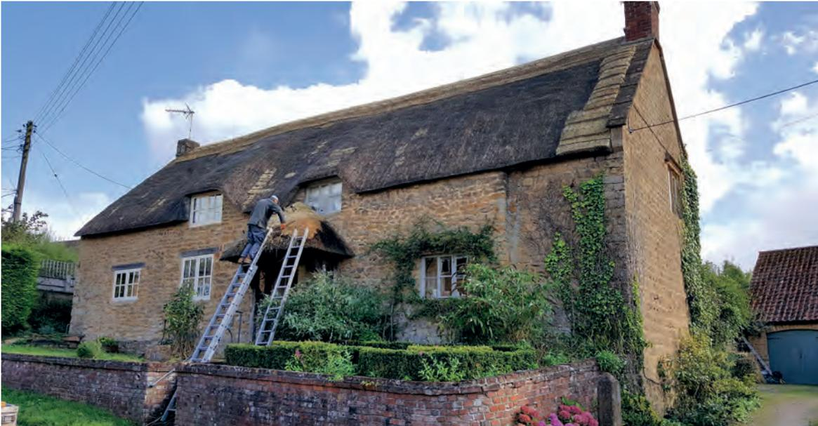
Patching thatch in discreet weathered areas will delay the need for complete spar coating for this Somerset house for several years.
