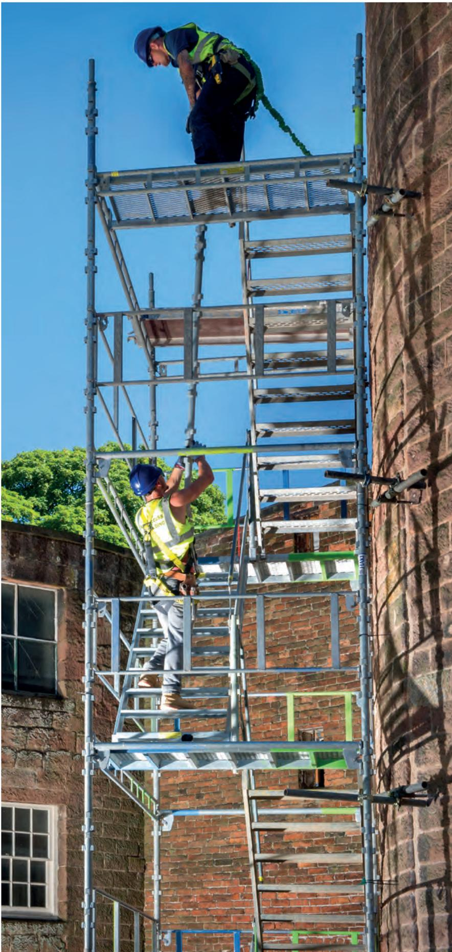
A modular access tower being constructed at Cromford Mill, Matlock: in this case the height to width ratio meant that fixings into the masonry were unavoidable.
