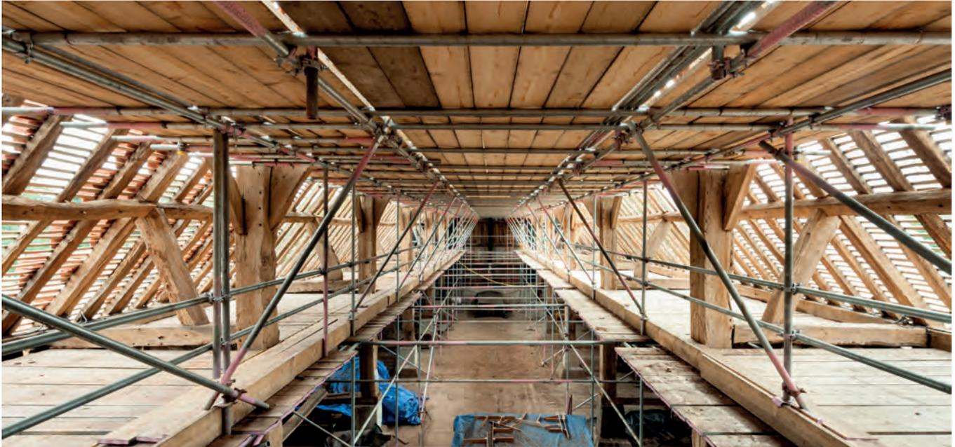
*A birdcage scaffold providing access for the repair of roof timbers from the inside: no fixings to the existing structure are needed because of the width. (All photos copyright Historic England)*
