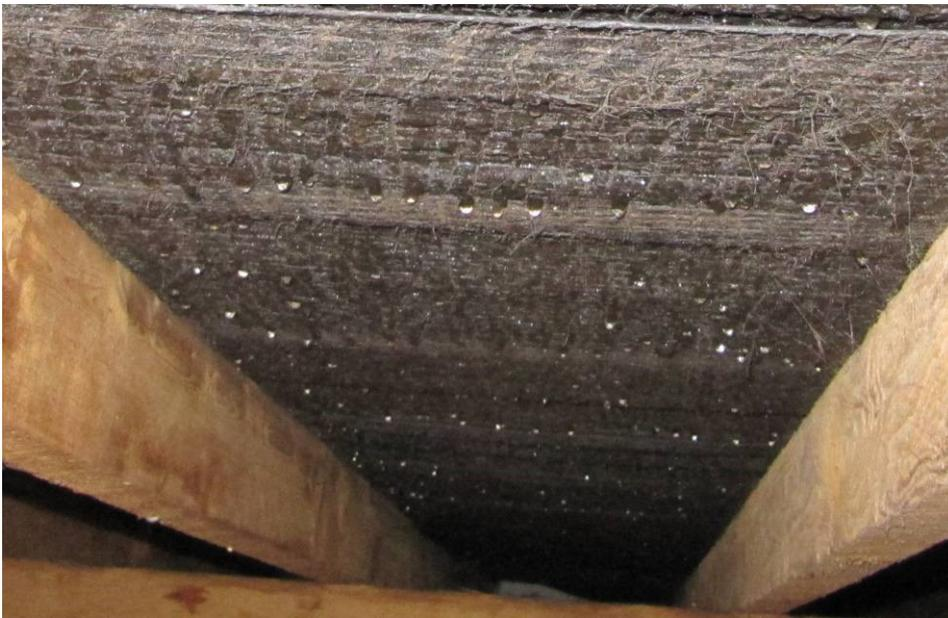
*Fig 113: A mouldy suitcase, drip marks on the floor boarding and condensation on the impermeable BS747 Type 1F underlay*
