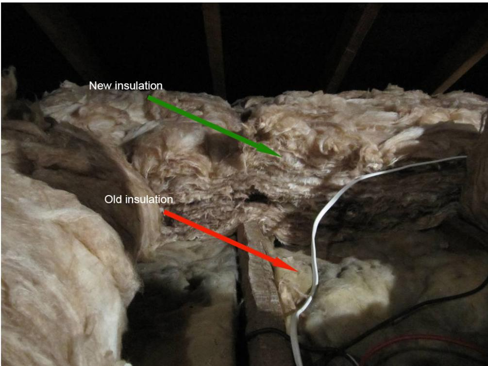
*Fig 111: Showing 100mm of glass fibre insulation, increased to 300mm in 2014*
