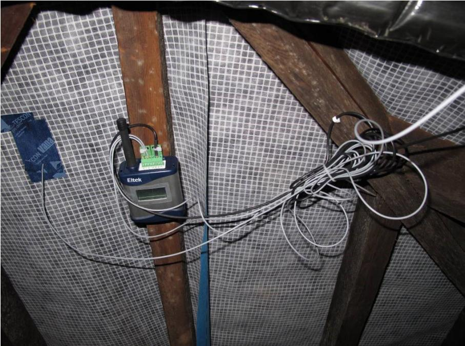
*Fig 48: The underlay was slit to allow sensors to be installed behind, then sealed with Tescon Vana tape*
