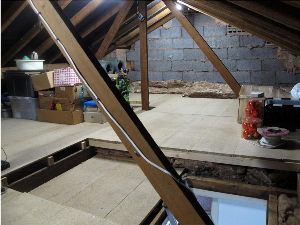
*Fig 110: Loft construction with an impermeable BS747 Type 1F underlay and a boarded floor*
