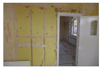
Fig. 75: The partition between the two rooms of the Victorian bedroom suite (F.04 and F.05), viewed from the south in early 2022. The wall has since been stripped back, the doorframe removed and the opening greatly enlarged. [Emily Cole © Historic England
