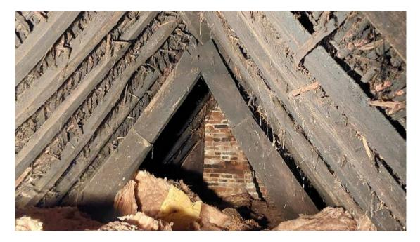
Figure 2a: Cruck truss 2 showing north face (note how each blade is made up of an upper and lower piece) (photograph Robert Howard)
