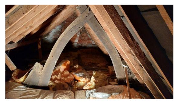
*Figure 2b: Upper section of cruck truss 4 showing north face (photograph Robert Howard)*
