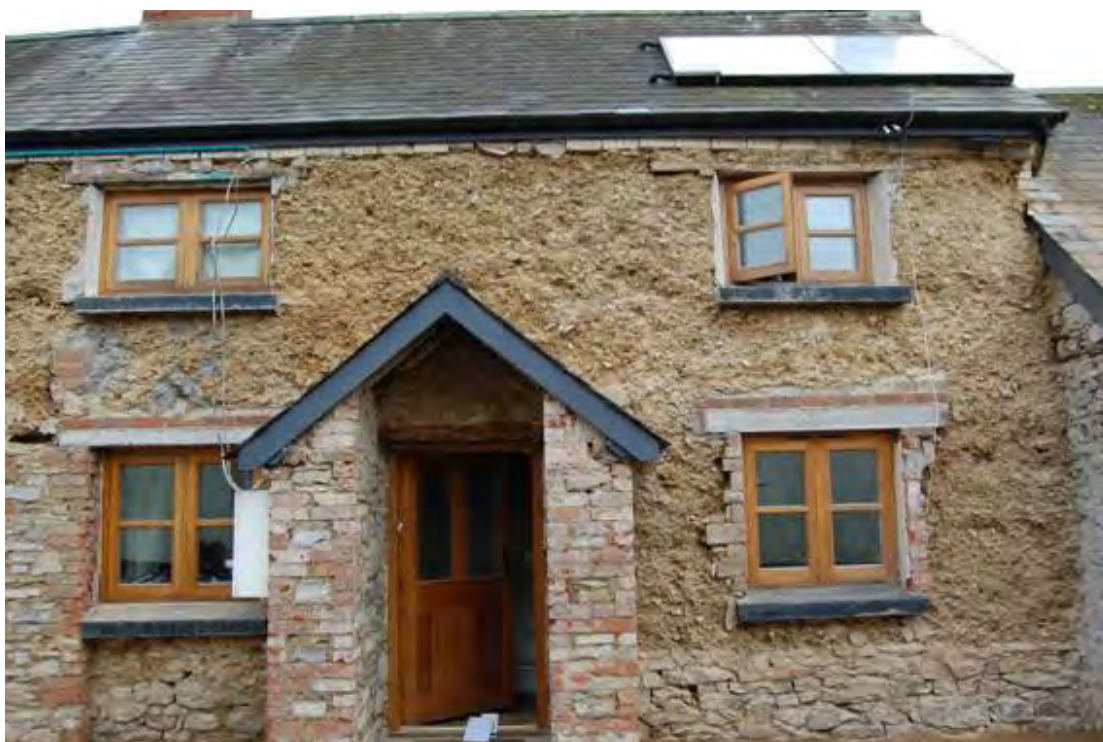
Figure 40. The Firs, Riddlecombe front elevation showing masonry buttress bottom left of frame.
