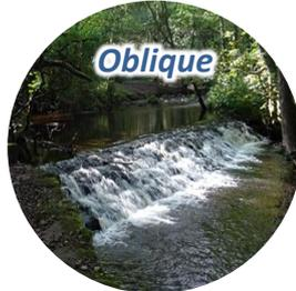
Weir spans the channel at an angle. Reduce the rise of water level at the least entrance during river spate due to increased length of crest. Can be combined with Curved.
