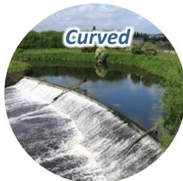
Weir takes horizontal arched form across channel. Increases length of crest and resists water pressure behind the weir by transferring the force to the river banks.
