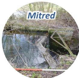
Weir forms a V-shape, the base of the V pointing up stream. Resisted water pressure similar to Curved.
