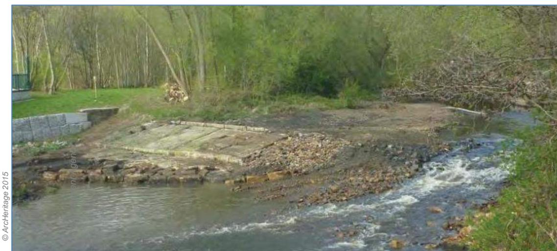
**Plates 31:** Ward End Weir following partial removal
