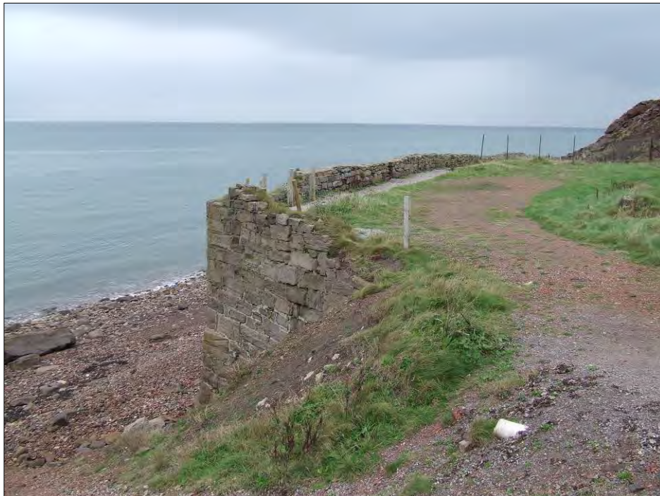
Figure 5.126 Remains of 18 th century sea wall erected to protect Saltom Pit Colliery, looking north.
