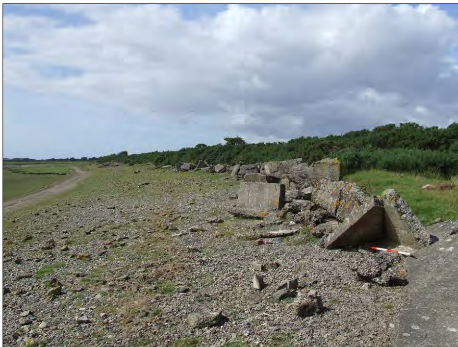
5.180 Second World War debris used as a flood defence on the Grune Peninsula, looking southwest (scale = 2m).
