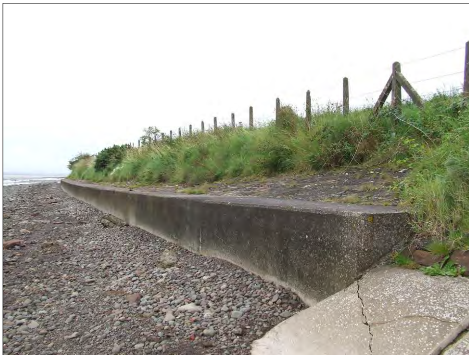
Figure 5.186 Shoreline west of Bowness-on-Solway showing a concrete and stone sea wall and upper shingle beach section.
