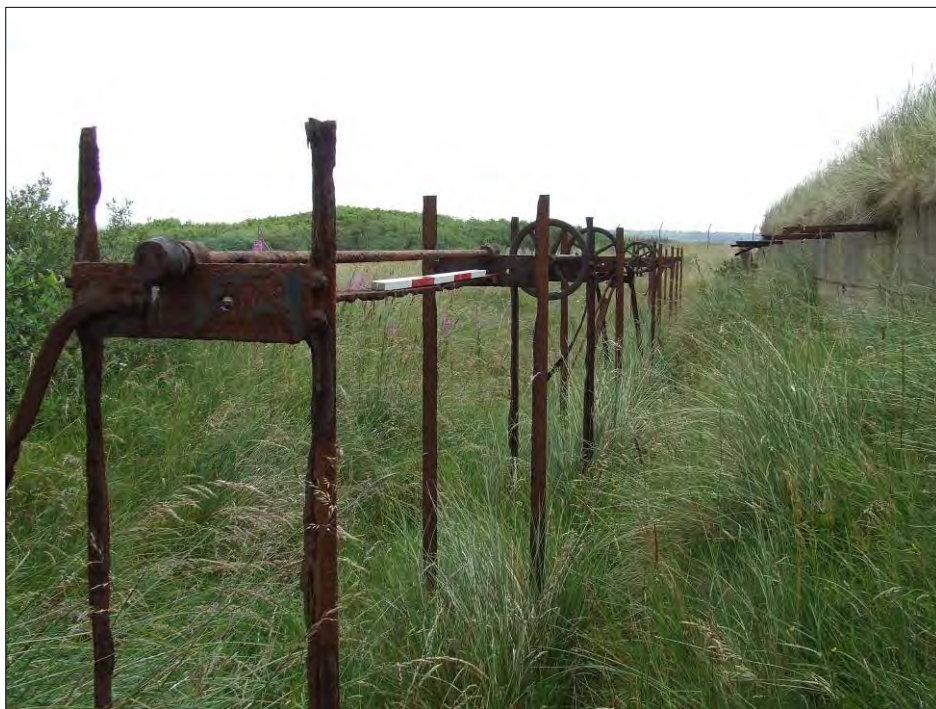
Figure 5.41 The southern embankment of the Second World War firing range at North Walney showing the concrete revetment and wrought iron mechanism for raising the targets.
