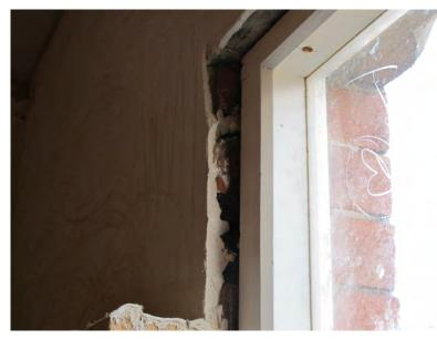
Figure 20: Varying thickness of the bonding coat of lime plaster
