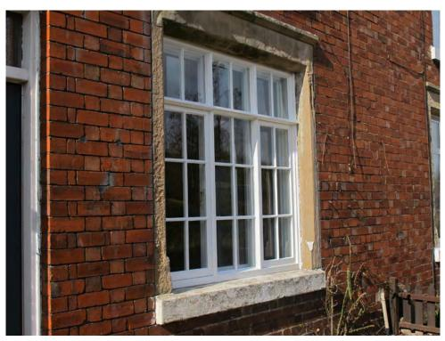
Figure 22: Restored casement window on the front elevation
