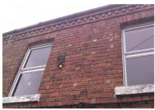
Figure 13: Plastic coated single glazed aluminium window on the rear elevation
