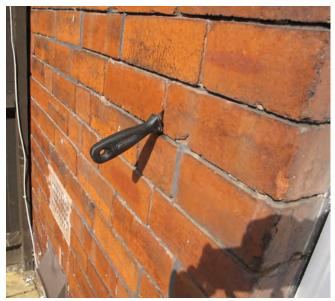
Figure 3: Deteriorated mortar joints
