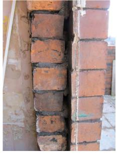
*Figure 5: Removal of the door frame revealing a cavity in the wall*
