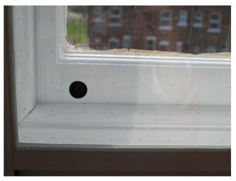
*Figure 25: Detail of the slim profile vacuum glazing*
