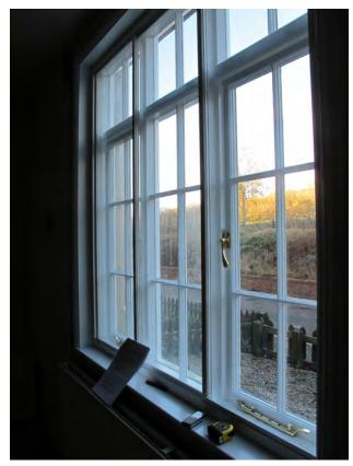
Figure 23: Secondary glazing on the casement window
