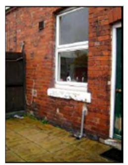
Figure 8: Irregularly laid paving slabs at the rear of the house channelling water to base of the rear elevation
