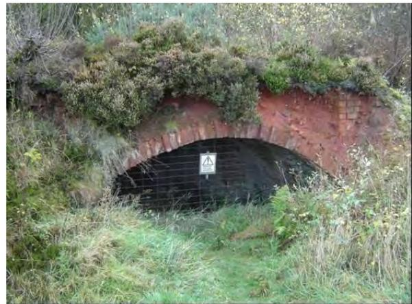
Plate 55 Whitakers & Sons brick kiln in former alum quarry, Peak Alum Works, built to produce bricks for Ravenscar, Scarborough and district
