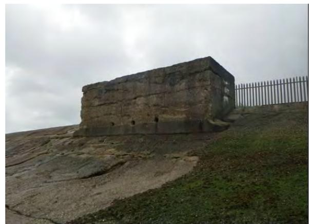
*Plate 206 Front of one of two WW2 Type 23 Lincolnshire variant AA pillboxes constructed on seawall, Grimsby, all embrasures blocked*
