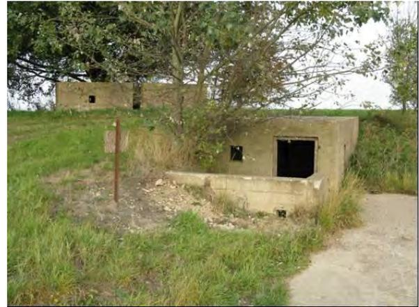
*Plate 212 WW2 variant pillbox apparently designed for reverse slope of seabank near Type 23 AA pillbox, Holbeach*
