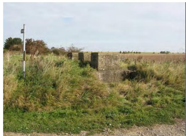
*Plate 213 Triple WW2 anti-tank blocks on a single strip foundation, Holbeach*
