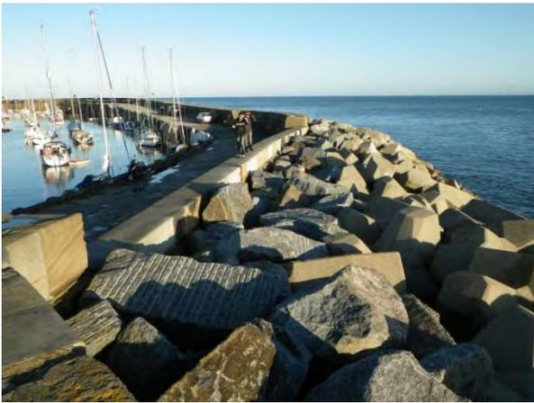
*Plate 123 Modern rock armour laid against east face of East Pier, Scarborough*
