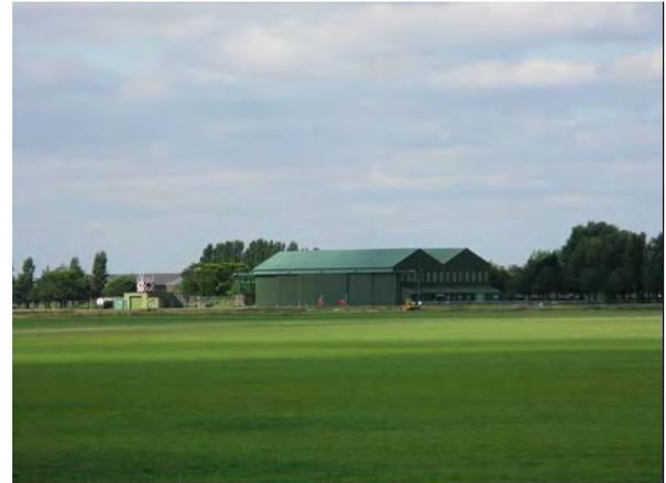
Plate 218 Rare 1930s two-bay 'No 4' hangar with side-opening doors, RAF North Coates
