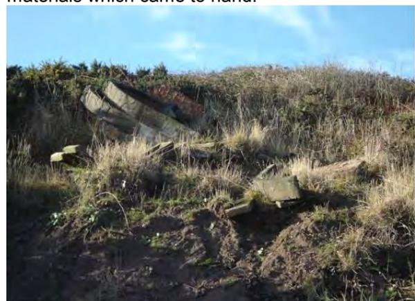
*Plate 168 Collapsed prefabricated segmental wall sections of WW2 Ruck machine gun post, Reighton*
