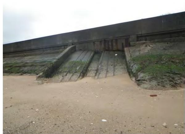
*Plate 142 Disused slipway of former shipyard north of the Fish Dock, Grimsby, blocked by later flood wall*
