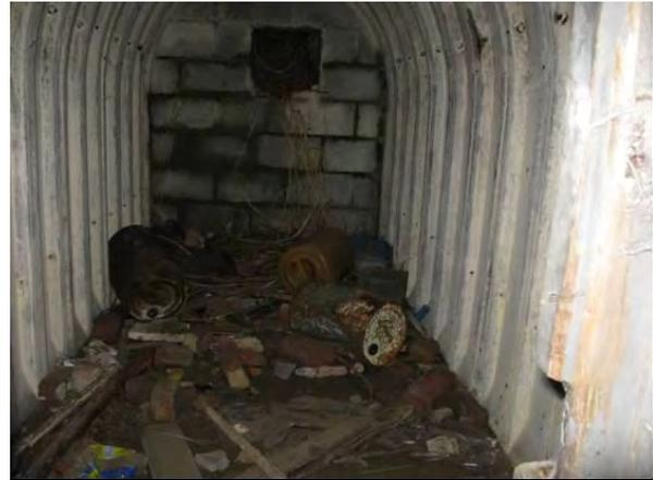
*Plate 221 Side chamber formed from Stanton shelter components, WW2 observation post, North Somercotes*
