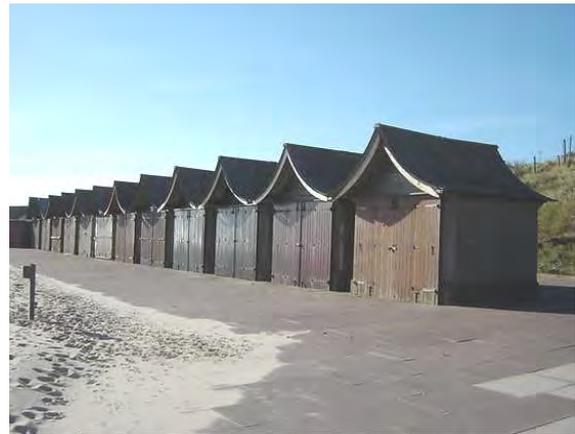
*Plate 315 Concrete and asbestos beach huts, Mablethorpe*
