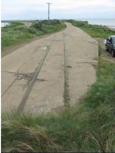
*Plate 179 Section of WW2 military railway embedded in later roadway, Spurn*
