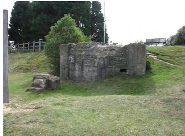
*Plate 204 WW1 trapezoidal pillbox with WW2 or later additions to support observation tower for RAF Theddlethorpe air gunnery/bombing range, Skidbrooke*
