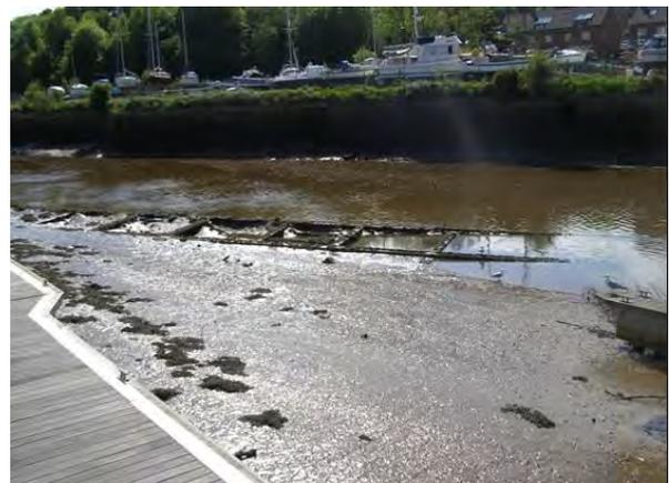
*Plate 112 Late 19th-century section of patent slipway, former Whitehall shipyard, Whitby*
