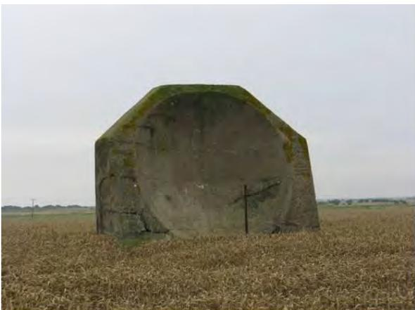
*Plate 180 Scheduled interwar concrete sound mirror with surviving microphone post, Easington*
