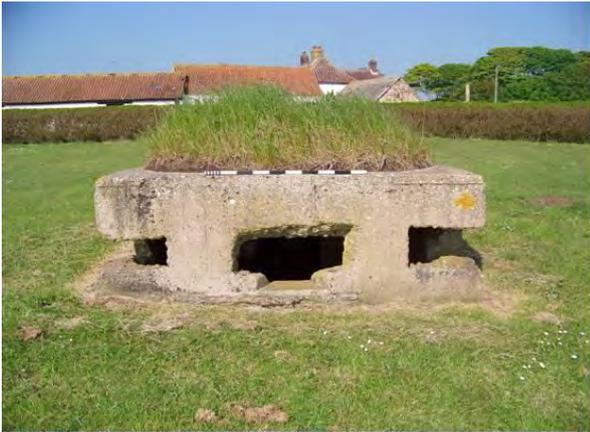
*Plate 182 WW1 square pillbox with WW2 machine-gun embrasures replacing smaller original single splayed opening, Auburn Farm*
