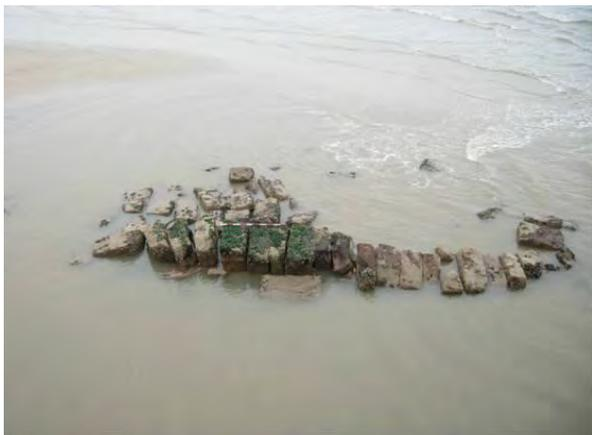
*Plate 130 Remains of the late 18th-century addition to the earlier timber North Pier, Bridlington, east of the present pier*
