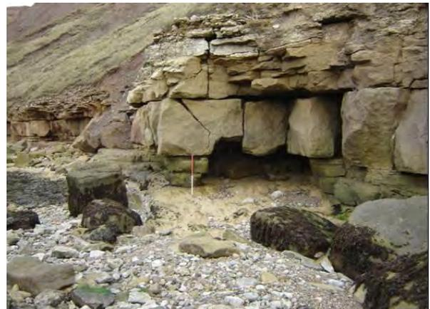
Plate 52 Pillar and stall quarrying, south side of Filey Brigg
