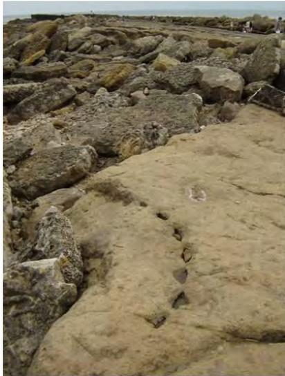
Plate 49 Line of wedge-pits for rock splitting, north side of Filey Brigg
