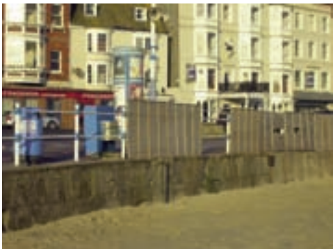
Figure 32 Since the early 19th century Weymouth has been protected by a solid sea wall. Sand now hides much of the walling, but some of the wall formed with large stone blocks is visible at the southern end of the Esplanade. In 1897, 63 sockets were fixed to the wall to hold flags. During the winter, fencing prevents sand from blowing up on to the Esplanade. [DP024379]
