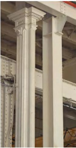
Fig. 52. Neoclassical iron columns cast in an industrial style inside Portsmouth Main Pumping Station No. 1 (1878, 2/201). A. Coats 2015. Reproduced with the permission of the MoD.
