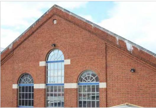
Fig. 54. East elevation showing the 1994 brick gable pediment to the extension of Bay 1 of Portsmouth Factory/100 Store (1903, 3/82), designed to appear similar to the original gable pediments. A. Coats 2013. Reproduced with the permission of the MoD.
