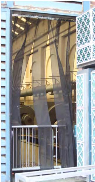
Fig. 60. Portsmouth Central Boiler House plastic door strips to keep out birds in summer (1907, 2/19). A. Coats 2013. Reproduced with the permission of the MoD.
