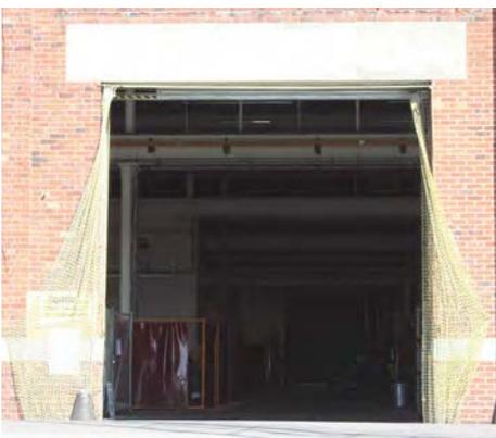
Fig. 57. Modified south entrance to Portsmouth Armour Plate Shop/No. 1 Ship Building Shop/Multi-functional Workshop (1867, 2/172) supplied with nets to keep out birds in the summer. A. Coats 2015. Reproduced with the permission of the MoD.
