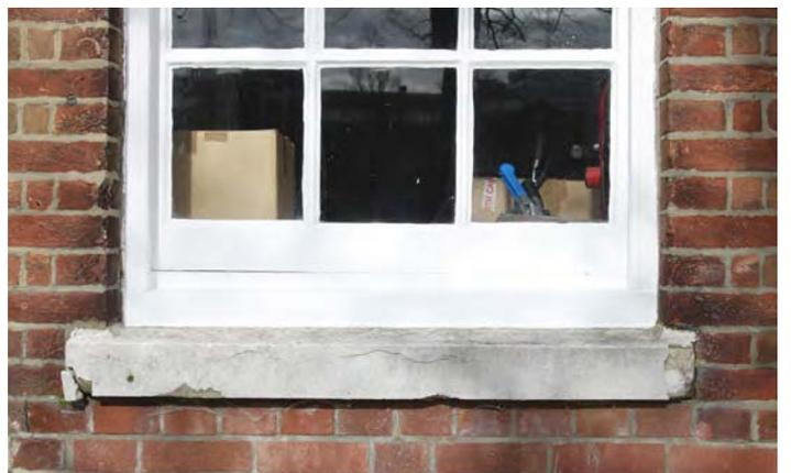
Fig. 39. Concrete sill showing deterioration, Portsmouth Storehouse No. 34 (c.1786, 1/149), modified after Second World War bomb damage. A. Coats 2013. Reproduced with the permission of the MoD.
