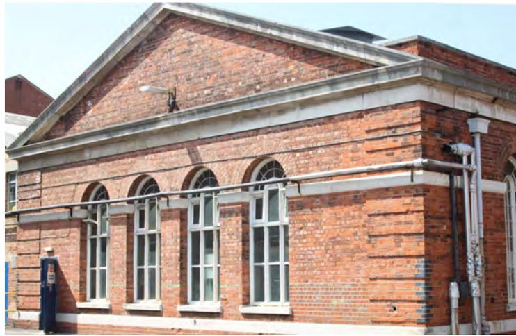
Fig. 53. Tall windows on the east elevation of Portsmouth Painters' Shop (1896, 2/191), to maximise natural light. A. Coats 2013. Reproduced with the permission of the MoD.
