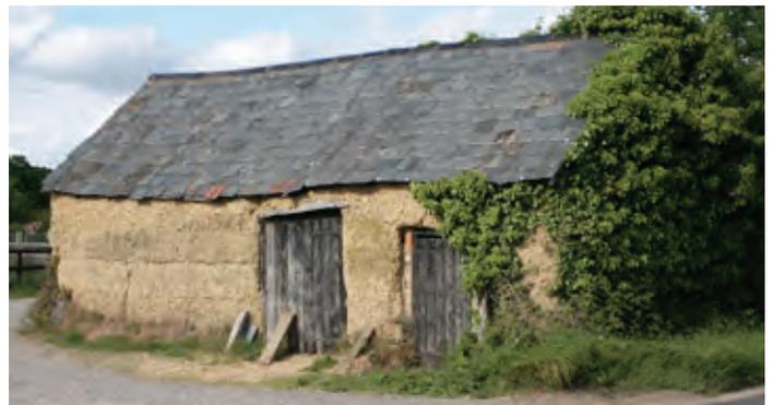
A small earth-walled building in the New Forest. The 'lifts', the phases of building up of the clay walls can be seen as horizontal bands of clay with slightly different textures and amount of small stones in the clay.
