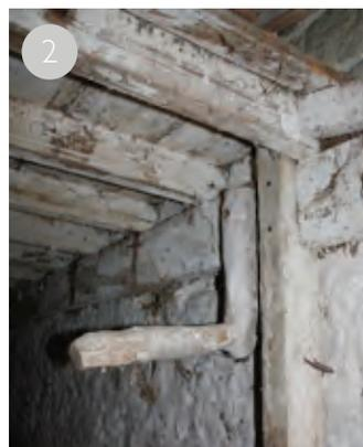
1 Lofted stables often have a hay drop along one side allowing hay from the loft to be lowered into hay racks on the ground floor. Here wattle hurdles have been used to block the hay drop.
