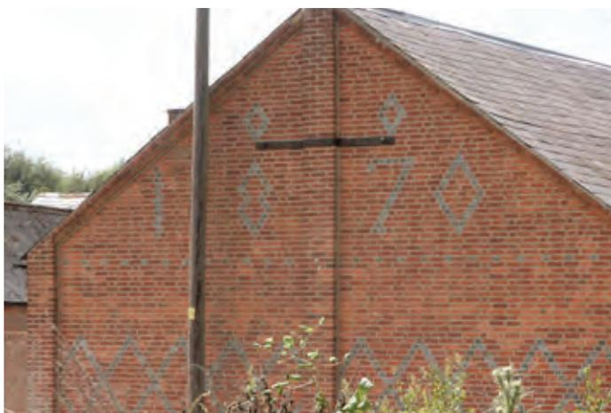
Late 19th century brickwork on an estate farm using burnt bricks to form lozenge patterns and to show the date of the building. In the late 19th century the use of machine made bricks became widespread. In this example a variant of Flemish bond is used but English bond made a return to favour, especially on estate-owned farm buildings. Photo © Bob Edwards
