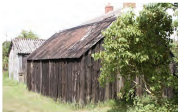
A small building on a New Forset smallholding clad in vertical round-faced boards. Photo © Bob Edwards
