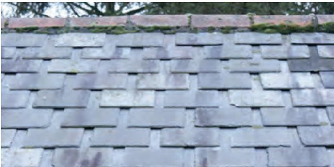
Welsh slate became readily available with the growth of the railways. Their lighter weight allowed for a reduction in the size of timbers need for roof construction. On estate buildings it is not uncommon to find slates being laid 'economically' to reduce the number of slates needed as so reduce the costs.
