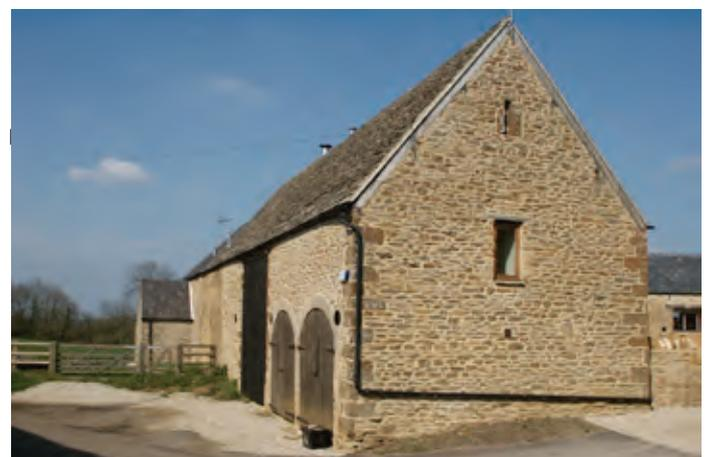
In regular courtyard plan farmsteads, as here in the Cotswolds, the cart shed often forms part of one of the ranges. Its function is identified by it having its openings on the external elevation of the range, facing onto the road which passes through the farmstead. Photo © Bob Edwards
