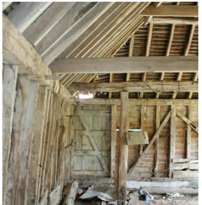
Shelter sheds usually provided shelter for cattle held loose in a yard but in the east of the region in particular open-fronted sheds could also be used to house tethered beasts. Any stall partitions have usually been removed but evidence of such use can survive including the presence of doors in the gable ends which gave access to a feeding passage along the back of the shed. Photo © Bob Edwards
