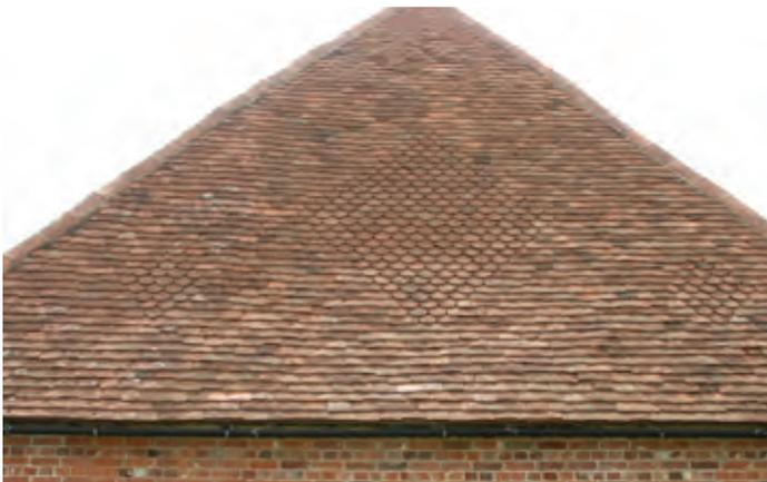
Plain clay tiles were being used to replace thatch in clay areas from the late 17th and early 18th century. Here the tiles include a pattern to the hipped end of a barn facing the roadside.
