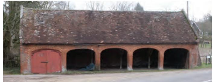
A brick-built cart shed in the South Hampshire Lowlands with one bay having doors so that small implements could be stored securely. Whilst most cart sheds were open-fronted, some examples retain evidence for having had doors to one or more bays in the form of pintel hinges in the posts. Photo © Bob Edwards
