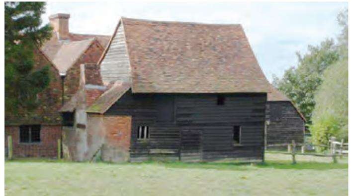
A rare survival of a detached kitchen to the rear of a High Weald farmhouse. Such buildings will often have smoke-blackened roof timbers to at least part of the roof and may have been partly floored. The stack at the gable end is a later addition. Photo © Steve Podd, FWAG
