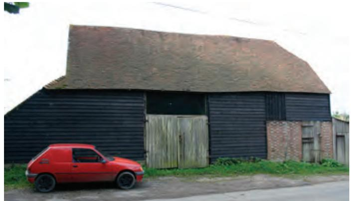
Stables could form part of combination barns from the medieval period. Here the stable element in the end bay has been rebuilt in brick. Photo © Bob Edwards
