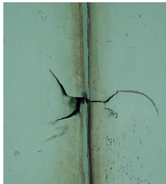
*Top:* Wind loading or thermal stress can cause a rectangular copper sheet, which is securely fixed at the edge to flex along the lines of folds which tend to be diagonal. Where the lines cross, additional stresses result in the star crack.
