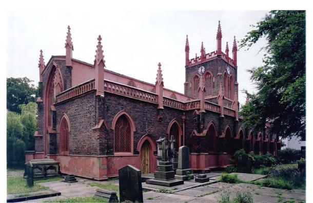
cast-iron elements. Closer inspection of the church reveals the novelty of its construction, with thin slate panels, originally sanded to take on the appearance of stone, encasing its brick shell at dado and clerestory levels. As with St George's, cast iron is also used for windows, tracery, parapet and pinnacles, and the interior is characterised by the decorative use of slender iron columns and delicate tracery.
