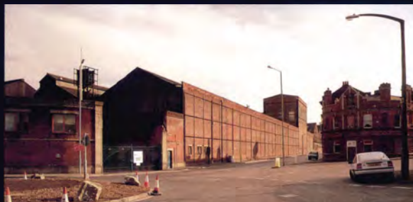
Fig 29 (top left) The large melting shop at Darnall Works, Darnall Road. Forming a single working area internally, the shop had 52 melting holes, contained in 12 stacks, 6 of which are seen rising through the roof. [AA022451]
