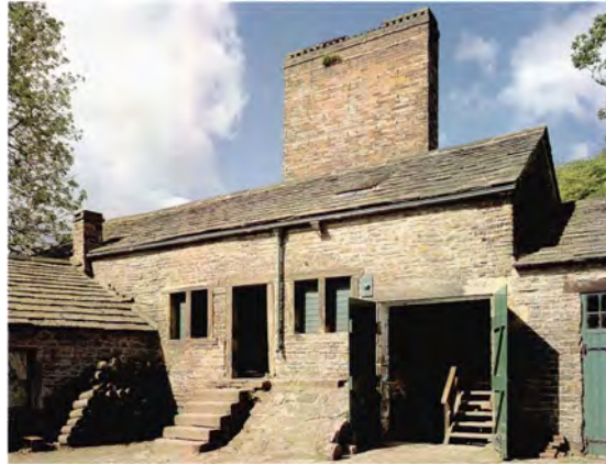
Fig 28 (far right) No. 35 Well Meadow Street: a mid- to late 19th-century works. In the foreground is the crucible stack, with lowered ventilation openings, iron strengthening to the base and metal ties in the upper wall. The small manufacturer’s house is situated beyond the workshop range and works entrance. [AA022450]
