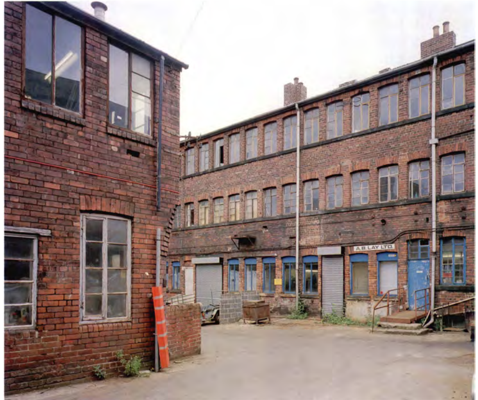
Fig 52 (right) A typical yard view in a Sheffield cutlery factory. The large number of flues served hearths inside the workshop. [AA022468]
