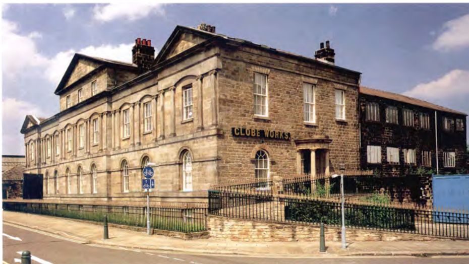
Fig 14 (left) Globe Works, Penistone Road: one of the new integrated cutlery factories built in the early 19th century. The Classical-style offices face the street and workshops are located at the rear. [AA022443]
