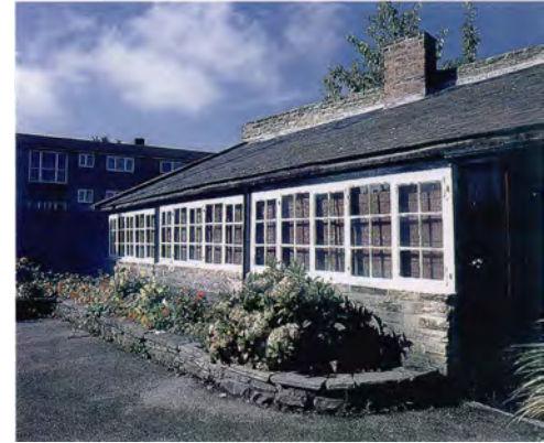
Fig 17 The file-cutting workshop at 11 High Street, Ecclesfield. The need for good light is indicated in the provision of long windows. Internal shutters gave security at night. [AA98/14081]
