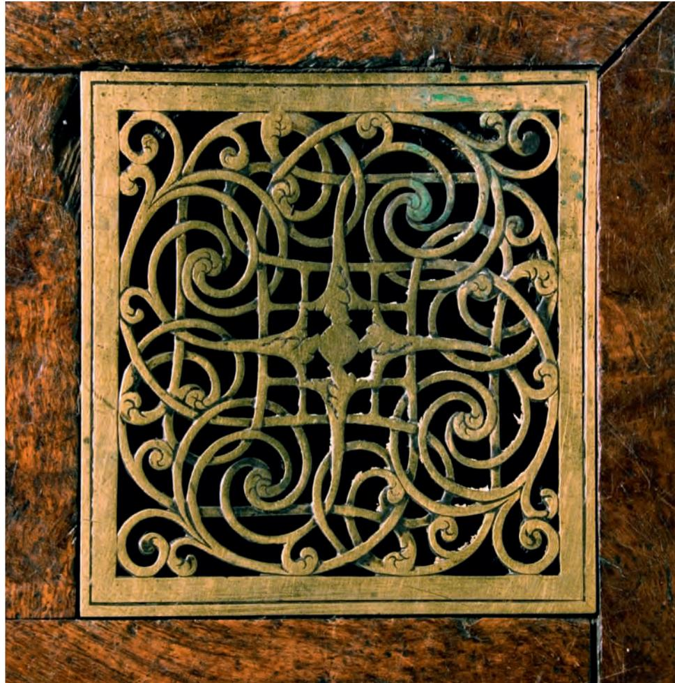
Wear and tear on architectural elements made from metals such as brass often incorporates damage to the metal and its surroundings from repeated polishing.
