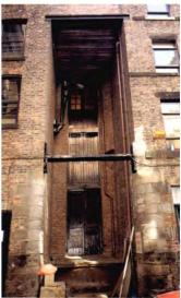
Fig 30 (opposite, top) Teagles and goods doors at the rear of 70–2 Portland Street (compare with the front elevation in Fig 29). [AA026864]
