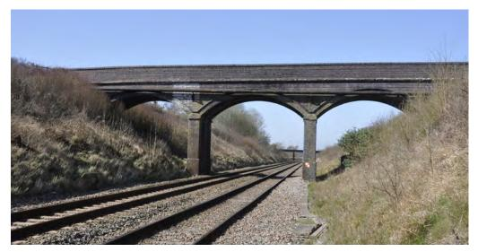
Fig 8: Accommodation bridge west of Chipping Sodbury tunnel (SWB 11132). A typical bridge on the SWB, the 'cut off' line to South Wales (with later attached pipes).
