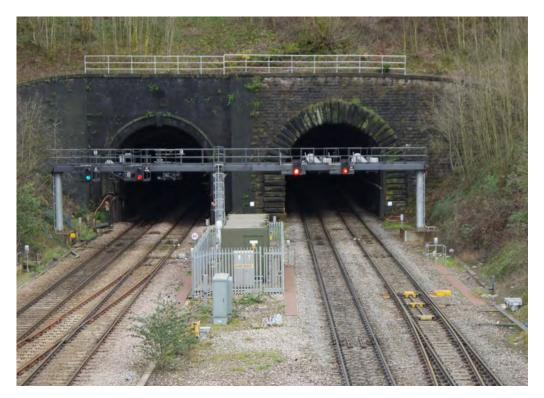
Fig 23: Newport (Stow Hill) Tunnel. The original (1848) portal and bore on the right, the left hand bore added 1911
