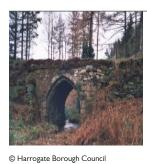
Medieval bridge, now crossed by a public footpath. The Butterton Bridge, Sawley / SITE NAME: structure is overgrown and decaying and there is danger of Warsill structural collapse. The bridge is now under new DESIGNATION: Scheduled Monument ownership and tenders have been obtained for repair, which is hoped to commence in 2020. CONDITION: Poor OCCUPANCY: N/A PRIORITY CATEGORY: F (D) OWNER TYPE-Commercial company LIST ENTRY NUMBER: 1004202 Contact: Giles Proctor 01904 601981
