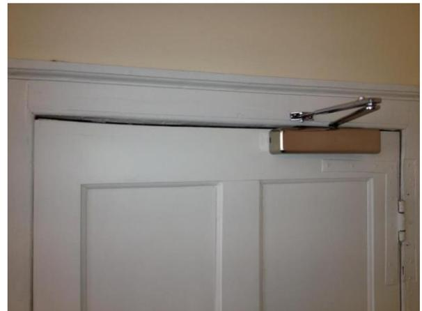
Lipping the top of the door or frame puts the repair in the most critical part of the door set during a fire. If the door can be raised by adjusting the hinges, the lipping can be applied to the bottom of the door.
