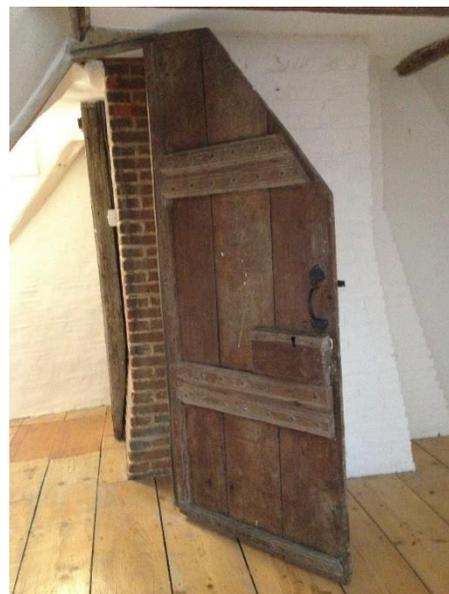
Ledged and braced doors are susceptible to warping from environmental changes and often have adjusted stops to accommodate the twist of the door.
