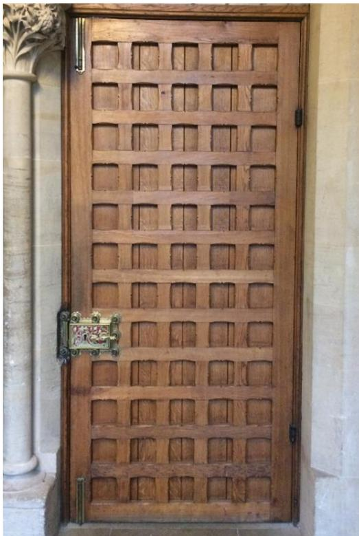
*Strap hinge bracing vertical planks*
