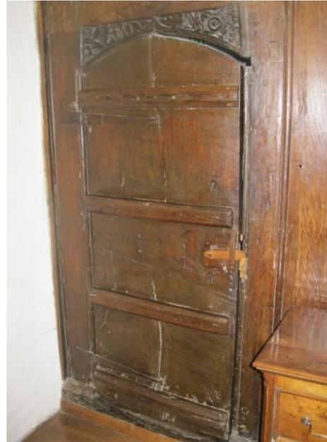
*Ledged door shaped to fit sloped ceiling. The ledges are wide enough to keep the door square*
