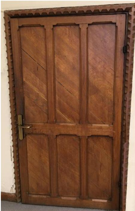
Although older doors and frames were not designed for fire protection, there are some cases where only minor modifications, as shown on pages 14-18 are required, particularly to panel doors to provide 20 or 30 minutes fire resistance in a fire test.
