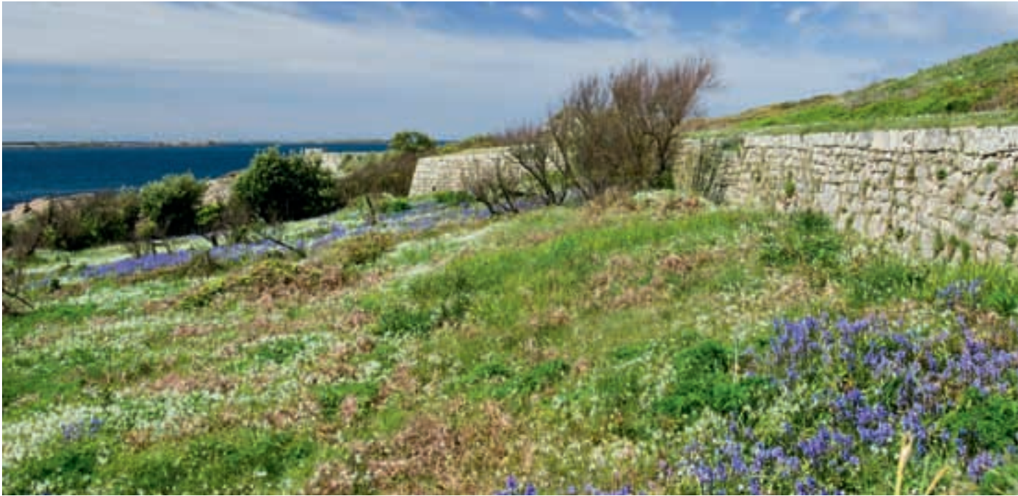
Figure 53 On the south side of the Garrison the stonework of the batteries is sometimes superior to the work in the intermediate walls. The stonework in this section, immediately to the east of Morning Point, is less regular than in the battery. In front were allotments once used by the soldiers of the garrison, but they are now home to wild flowers. [DP022458]
