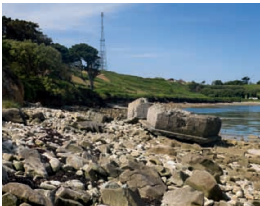
Figure 2 Once part of the circuit of Second World War defences, the pillbox at Pendrathen has succumbed to the rapid erosion of the coastline and now sits on the rocks. [DP085375]
