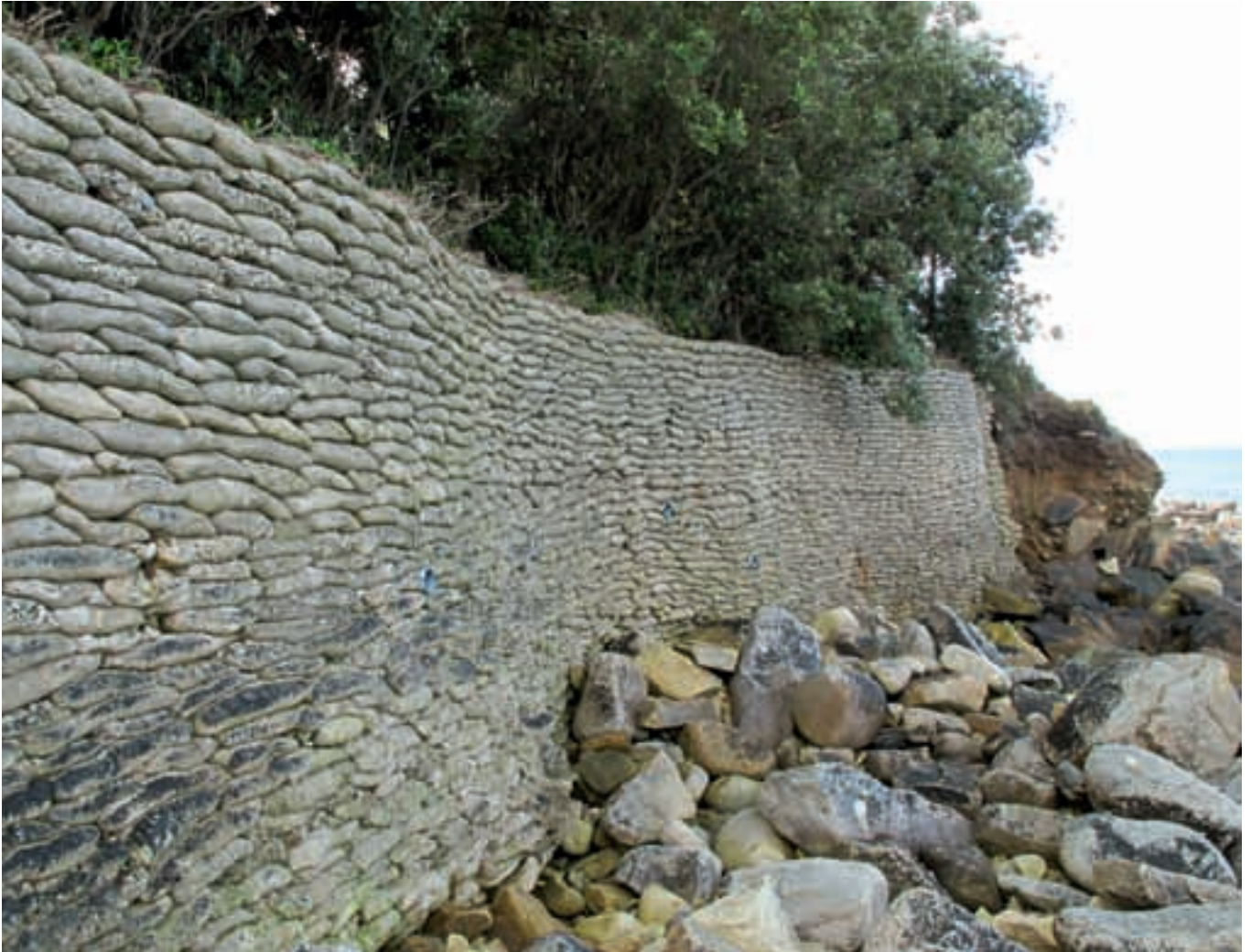
Figure 90 At King Charles' Battery at the north of the Garrison a previous cavern undermining the cliff has been reinforced by concrete sandbags to prevent its collapse. [DP086023]
