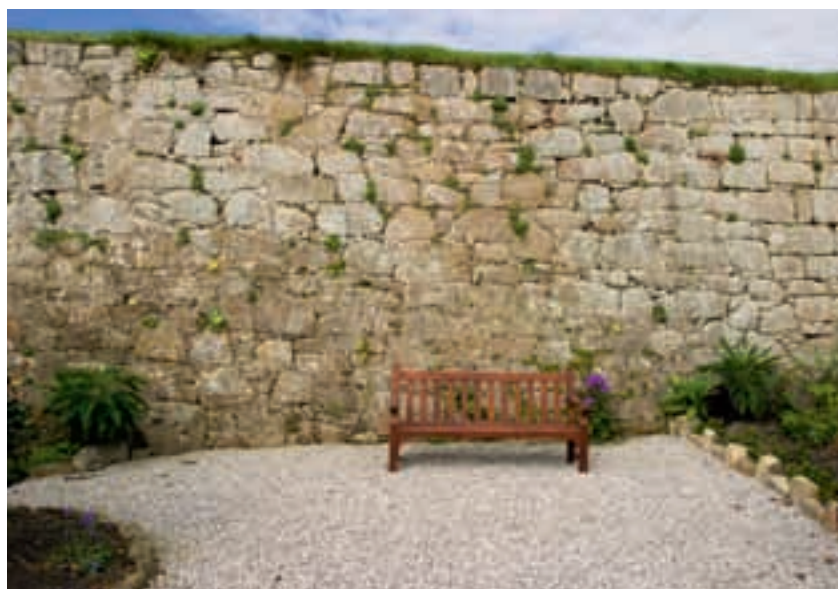
Figure 19 (right) The earliest stage of the Garrison Walls, dating from the 1590s, is easily recognised by large irregular stones with small packing pieces used to the joints. At the far right of this photograph is more regular stonework where the rebuilt Garrison Gate of 1742 was inserted into the original walls. [DP022358]
