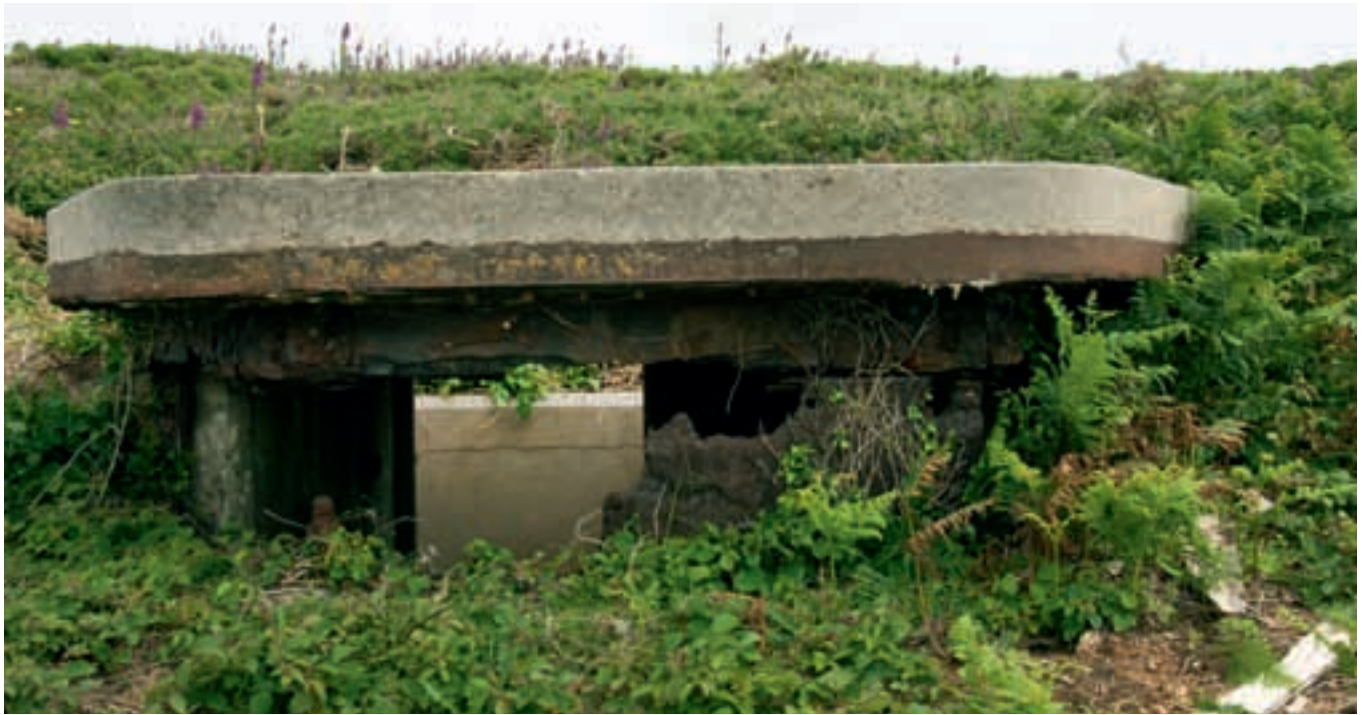
Figure 69 On the hillside between the 18th-century Woolpack and its c 1900 successor above, this small Position Finder Station set into the ground would have identified targets and tracked their movement with the help at night of the DEL. [DP085220]
