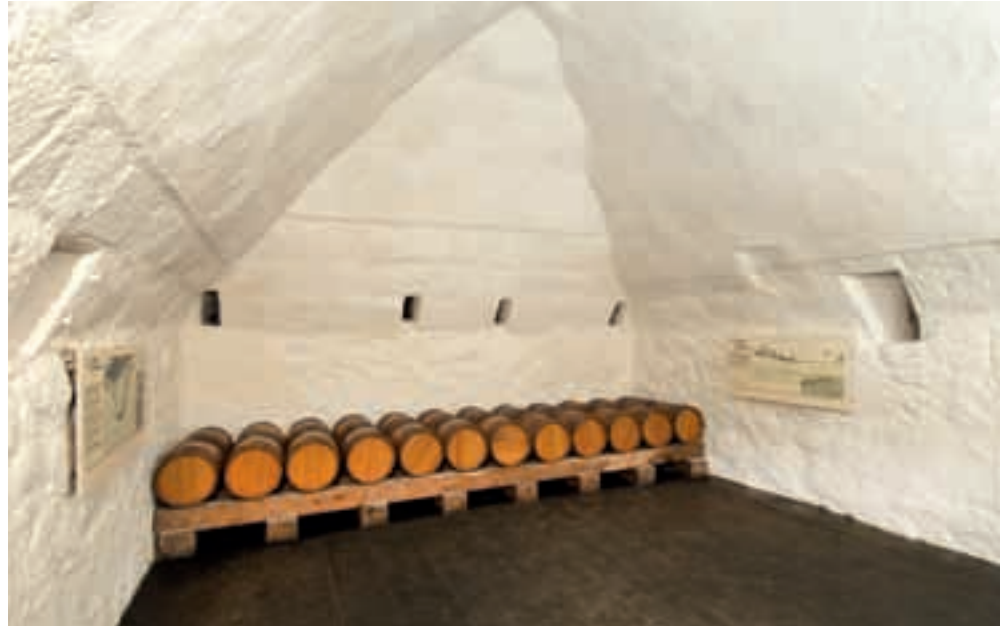
Figure 20 Probably dating from the 1620s, though with considerable later alterations and reconstructions, the magazine near the entrance to the Garrison has a strong vaulted ceiling and very thick walls. These are only pierced by small openings to provide some ventilation and to admit a little light from lamps or candles kept safely outside the structure. [DP085223]
