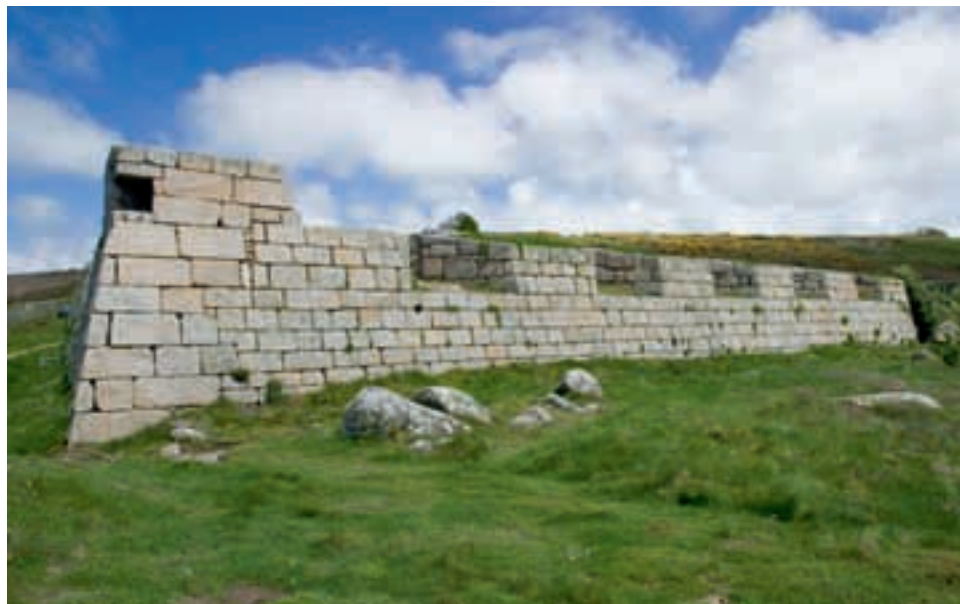
Figure 53 On the south side of the Garrison the stonework of the batteries is sometimes superior to the work in the intermediate walls. The stonework in this section, immediately to the east of Morning Point, is less regular than in the battery. In front were allotments once used by the soldiers of the garrison, but they are now home to wild flowers. [DP022458]
