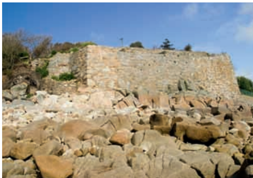
Figure 85 Lower Benham Battery bears the marks of repeated repairs, including one resulting from a collapse in 2004. This battery at the western end of Porthcressa Beach was designed to prevent invaders getting round the end of the Garrison Walls as they existed in the late 16th century. [DP022418]
