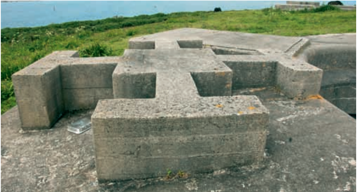
Figure 75 On the aprons of the c 1900 Woolpack Battery are the bases for the twin masts for the 'RACON' installation established at the Woolpack Battery in 1943. [DP085199]
