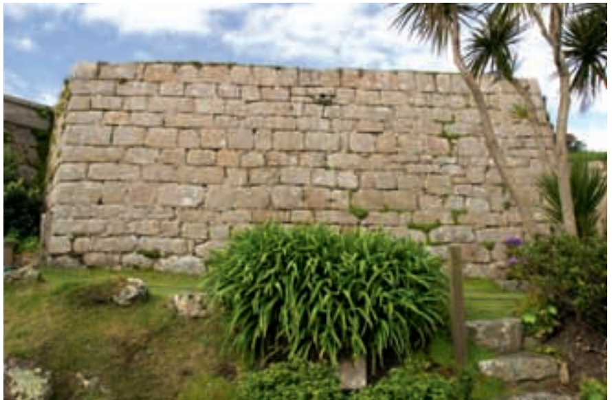
Figure 48 Higher Bastion, also known as King George's Battery, is immediately to the south of the Garrison Gate. The site of a bastion since the 17th century it was rebuilt in 1744–6 in neat, large blocks and with projecting spouts. [DP022362]
