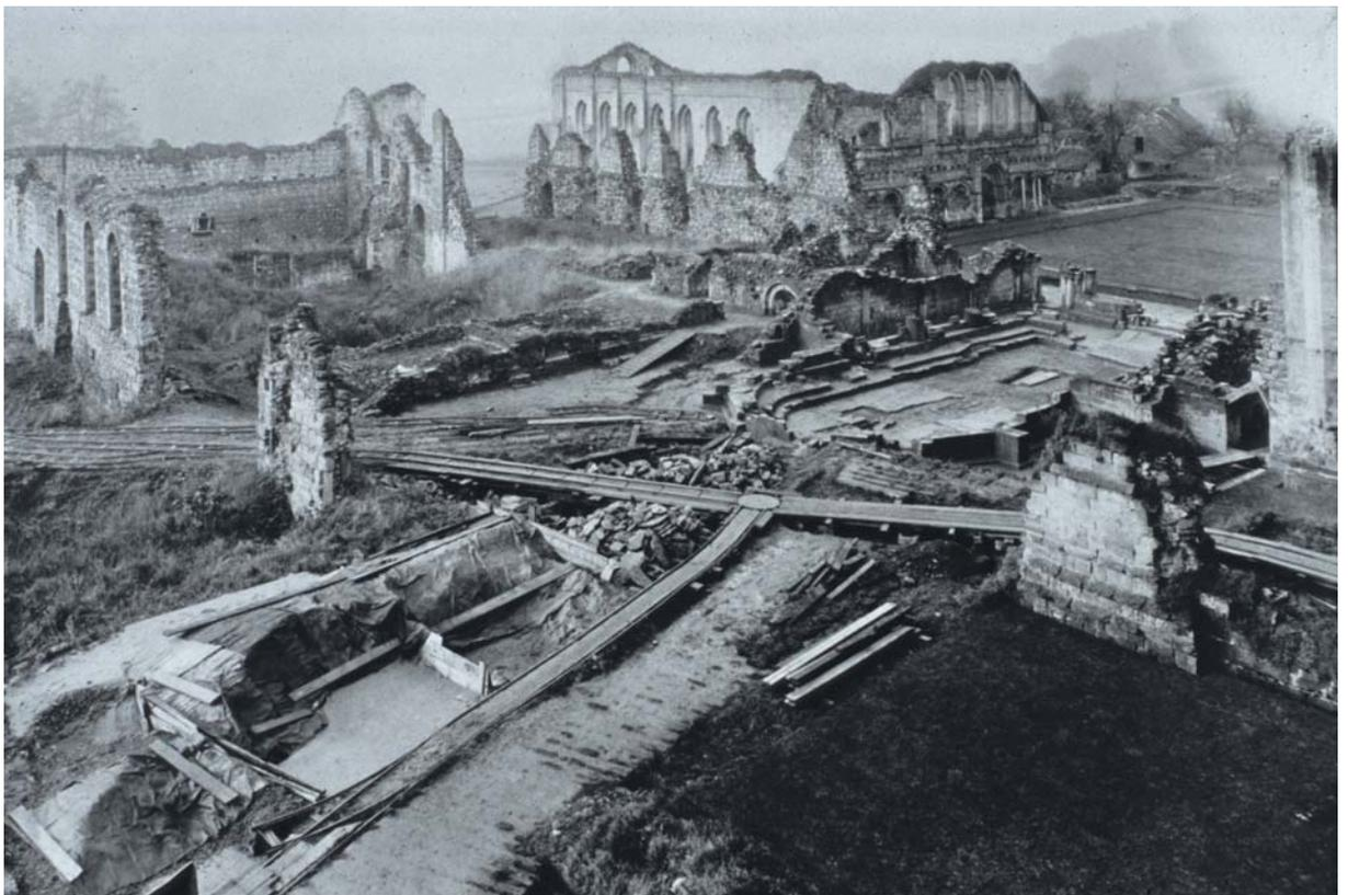
Site clearance in progress at Rievaulx Abbey in about 1921. Such was the scale of the works that a light railway system was used to transport spoil from the site.
