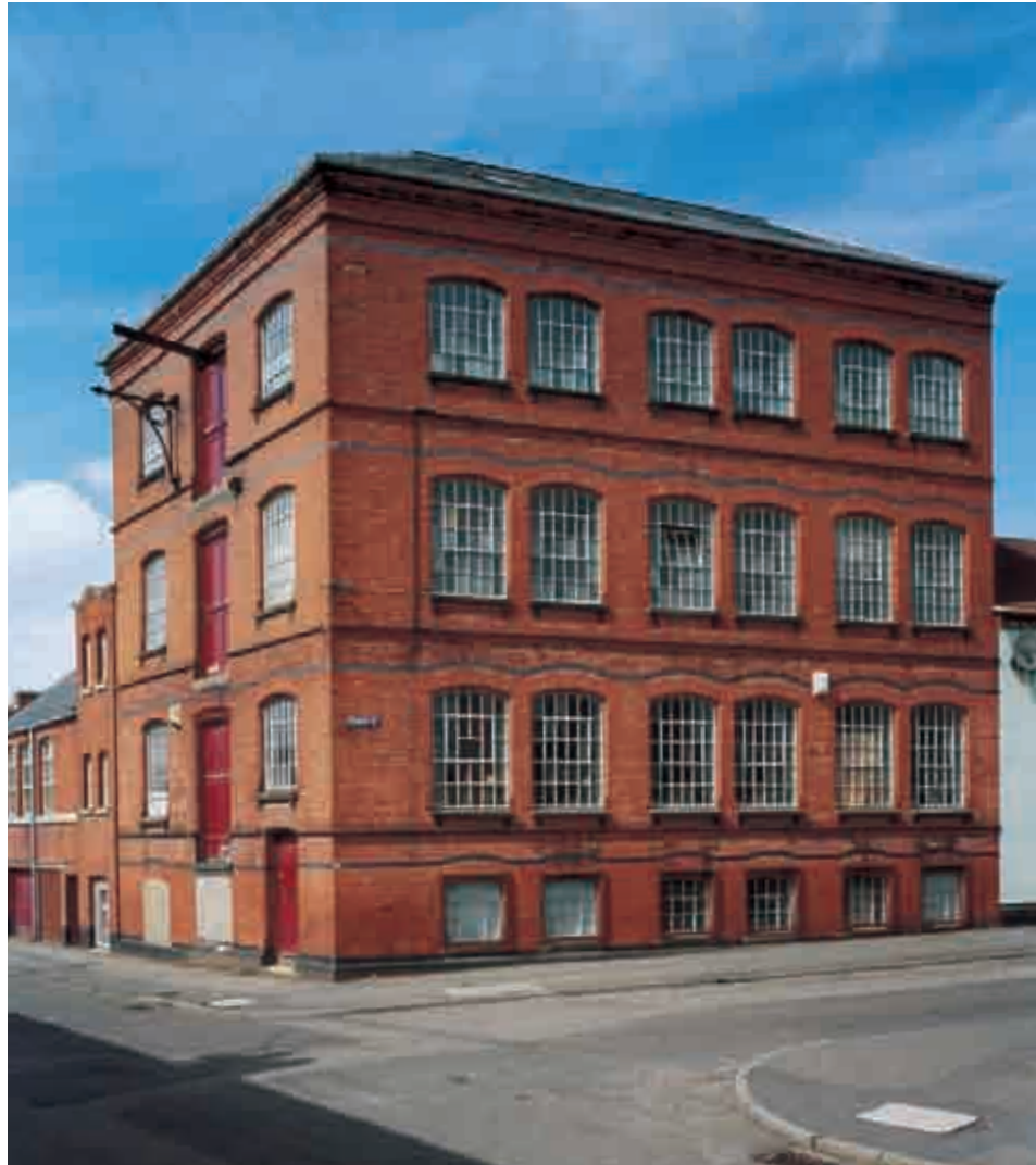
Fig 3 Although no longer used for its original purpose, this factory on Crabb Street in Rushden is well cared for and retains most of its original features, including its crane, loading doors and windows. It was built about 1887. [BB013242]
