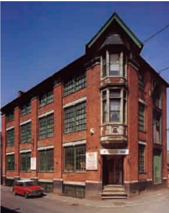
Fig 30 The Havelock Works of Kettering Co-operative Boot and Shoe Manufacturing Society was built in 1890: note the relief and motto on the oriel window. Factories often occupied corner sites to obtain maximum lighting. In such cases it was common for the corner bay to contain a prestigious entrance leading to offices, which is the arrangement here. [BB001992]
