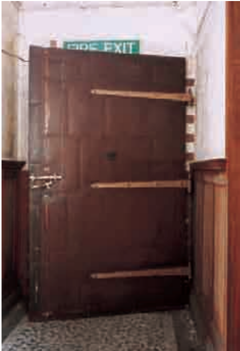
Fig 37 A Mather & Platt fire door in G T Hawkins's Northampton factory, separating the office suite from the production floor. It was installed in 1915. [AA044154]
