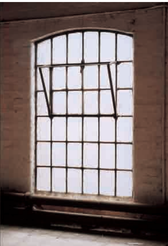
Fig 55 A typical cast-iron window which says 'factory' to us all, lighting the first floor of the former Hawkins's factory on St Michael's Road, Northampton. One of the most effective ways of safeguarding the character of factory and workshop buildings is to retain these original windows. Note the low sill, the opening hopper and the hot-water heating pipes. [AA044156]
