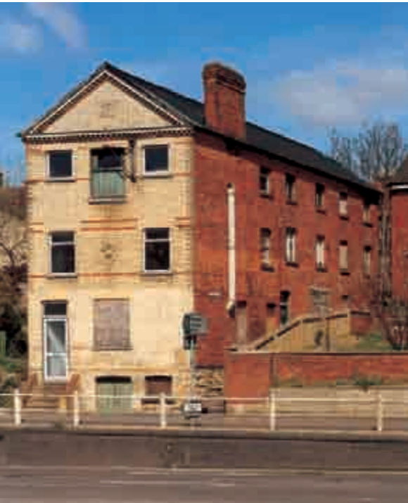
Fig 53 The boot and shoe factory at 83 High Street South, Rushden, was built in 1874. A two-storey house at the front of the building, served by a broad stack, is sandwiched between the basement and upper floor of the factory. This ingenious idea, prompted perhaps by the steeply sloping site, does not seem to have caught on. The entire building is now in residential use. [BB001997]
