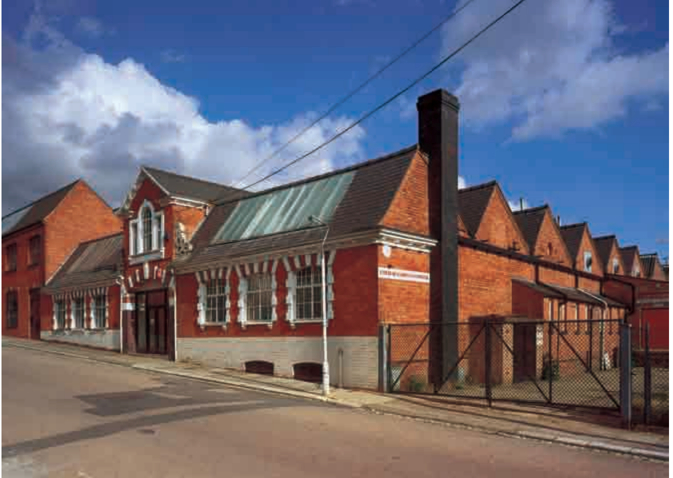
Fig 35 A Lee's Enterprise Factory was built on Bective Road, Northampton, in 1902. The north-facing slopes of the sawtooth roofs contain skylights. [BB013273]
