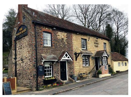
Many cottages in Graffham, Washington and Fittleworth are built entirely of carstone, laid to course in brick-sized blocks. It is also widely used as rubble walling stone, and occasionally as cobbles. Galleting, using small chips of carstone placed in the mortar between dressed Malmstone and Hythe Sandstone, is evident in many house and cottage walls in Midhurst, Pulborough, Storrington and Washington.
