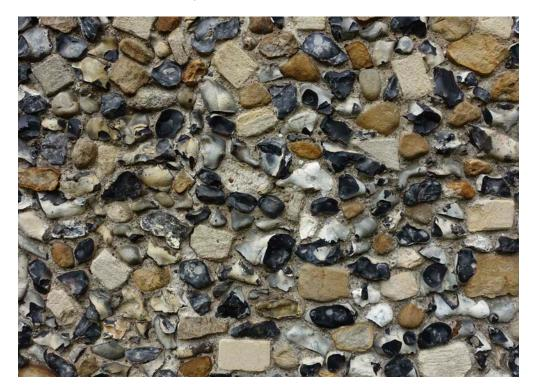
Figure 36: Church of All Saints, Melbourn. Quarry Flint nodules, blocks of Lincolnshire Limestone and brown quartzite and Quaternary pebbles and cobbles. Figure 37: Church of All Saints, Melbourn. Knapped Quarry Flint nodules with varieties of Lincolnshire Limestone, Melbourn Rock and Quaternary pebbles and cobbles.
