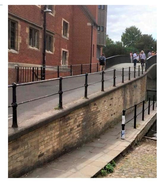
Figure 45: Garret Hostel Bridge, Cambridge. York Stone paving slabs.
