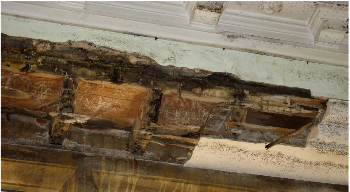
**Figure 8: Collapsed plaster due to water penetration via lead parapet gutter (image © Historic England)**
