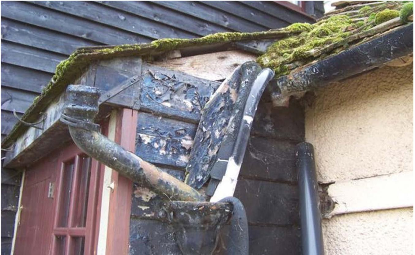
**Figure 5: Defective rainwater gutters and downpipes (image © PCA)**
