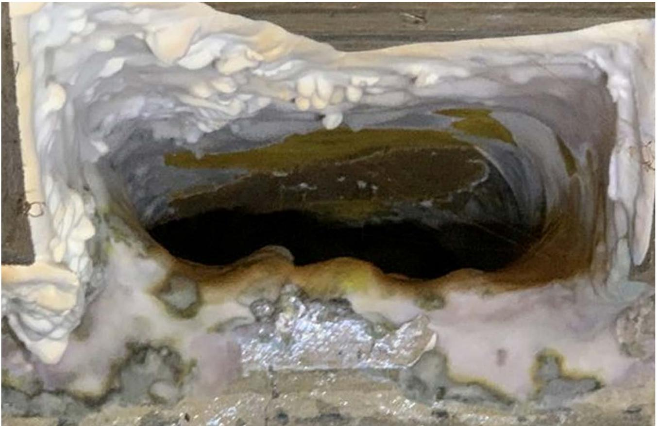
**Figure 6: Dry rot under a suspended timber floor (image © RICS)**
