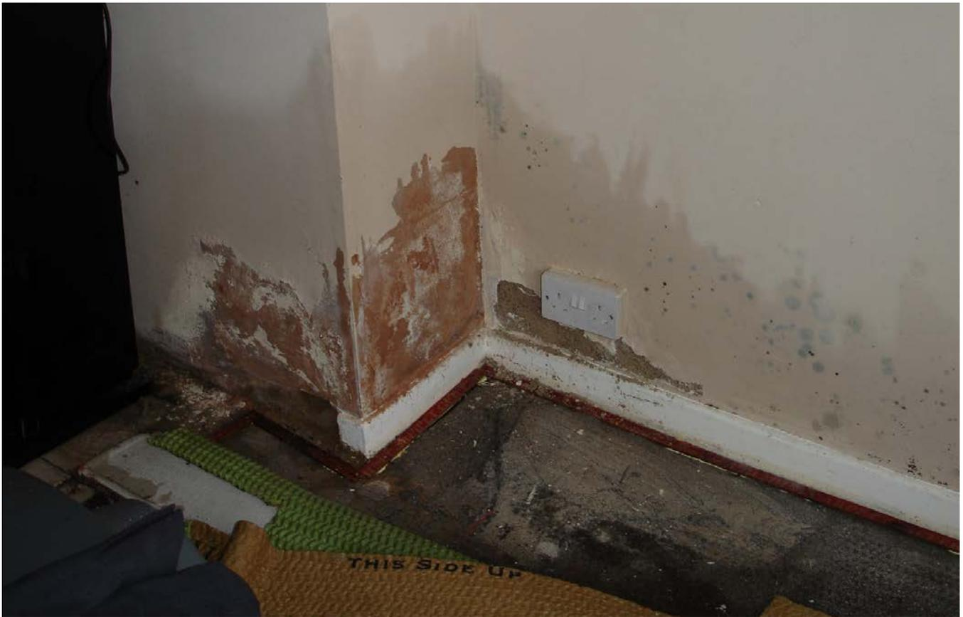
**Figure 4: Elevated moisture in a wall (image © PCA)**
