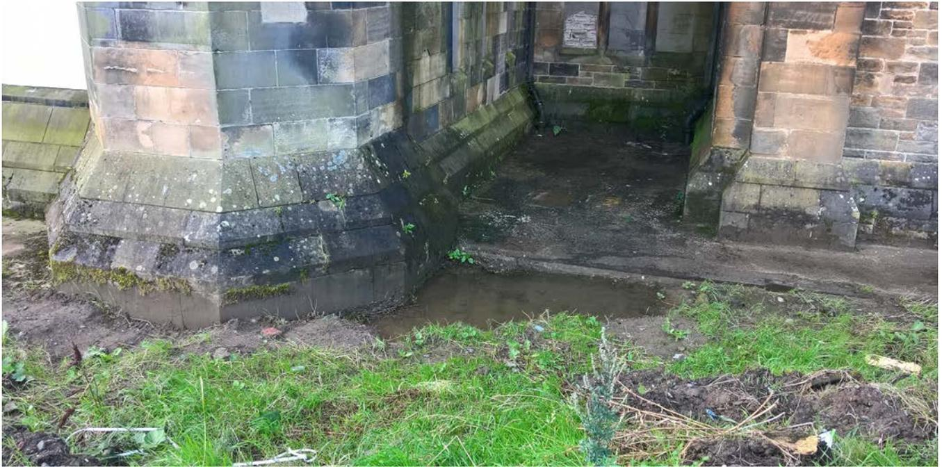
**Figure 3: Defective rainwater disposal (image © Historic Environment Scotland)**
