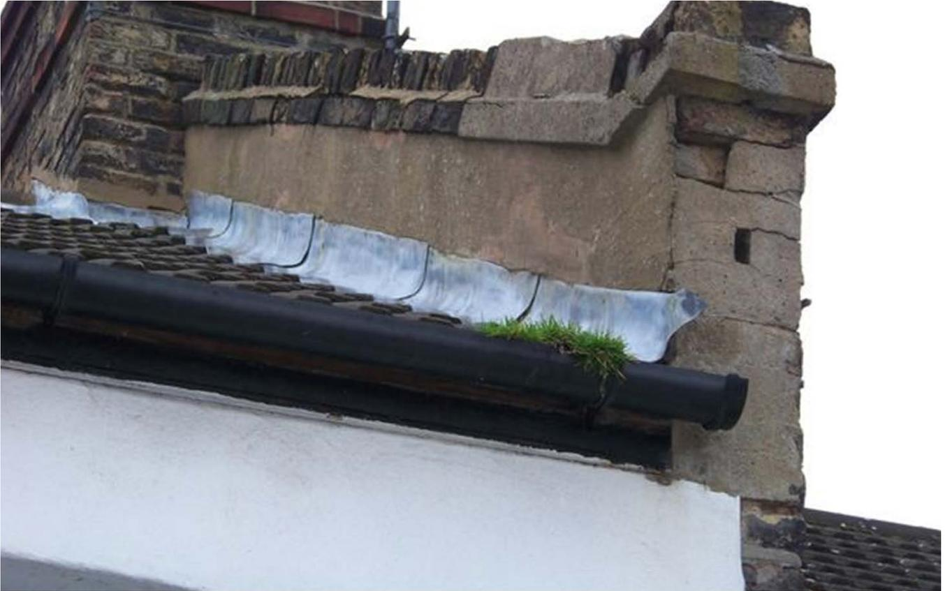
**Figure 1: Parapet wall in poor condition (image © PCA)**
